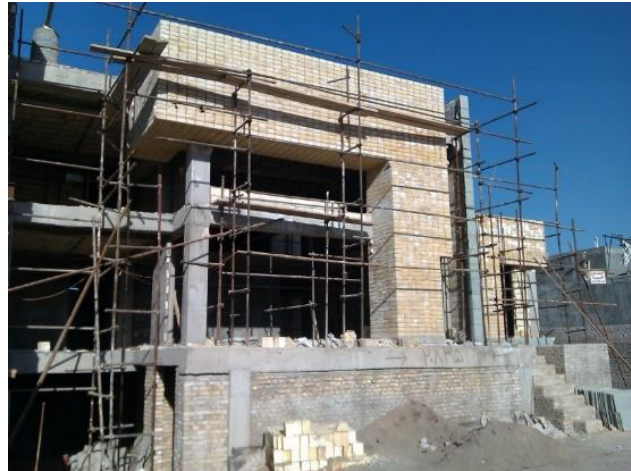
Figure 166, a typical house in Yazd with reinforced concrete structure, Daei house, designed by M. Mostafazadeh, photo from Mostafazadeh
