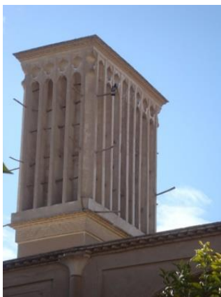
Figure 142, Tehrani House 4 sided wind catcher Photo and plan of wind catcher and the front Eivan, facing the pool and garden in the courtyard
