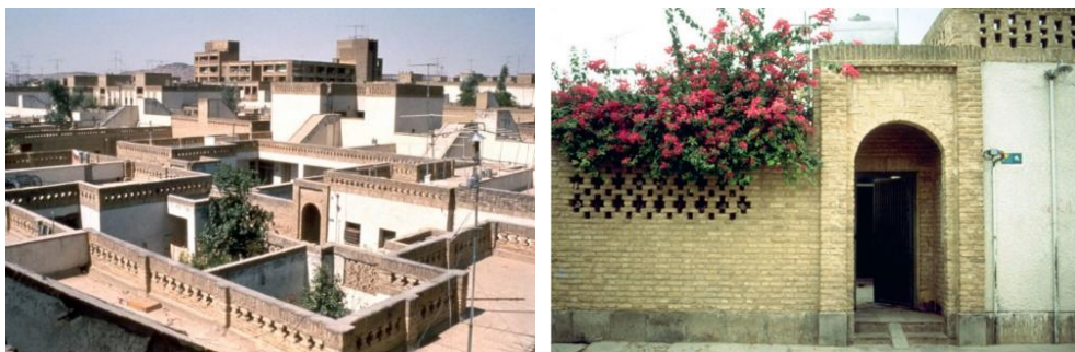
Figure 30, Shushtar New Town, central courtyards and brickwork grilles assisting in better air ventilation, Source: (DAZ 1986), ©Kamran Adle
