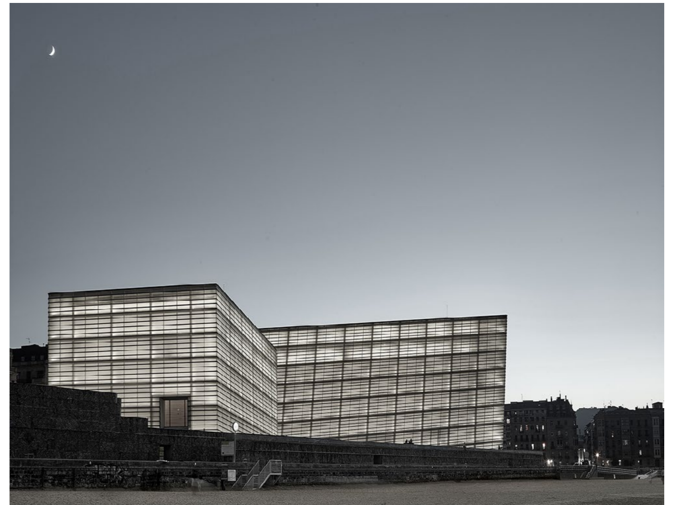
III. 17 Facade of Kursaal Congress Centre
