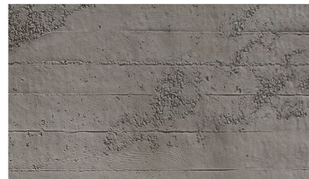
ORTBETON, WU - BETON
