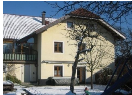
Abb.09: W6, Zubau(1990), WSW-Fassade
