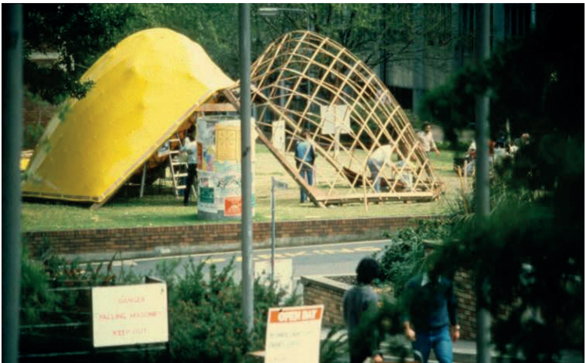
Fig. 2.29 LSRU Grid shell pavilion assembled and erected, 2nd part before covering [27]
