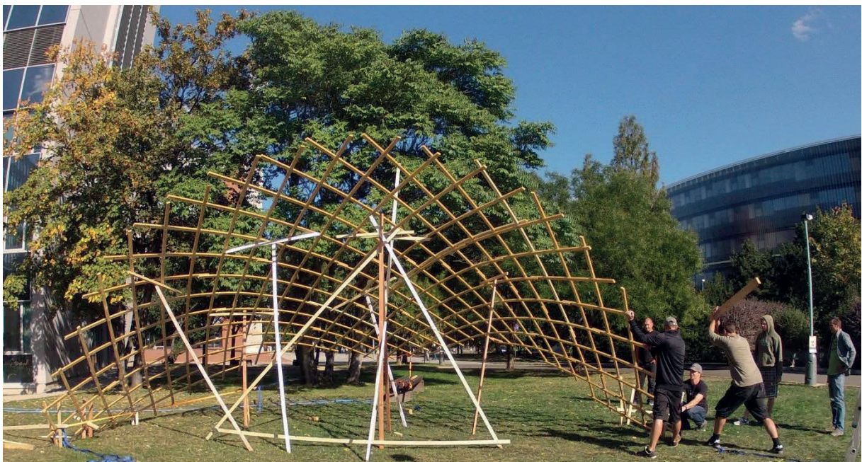
Fig. 6.4 Erecting procedure – Supported final shape anchoring [by author 28.9.2015]
