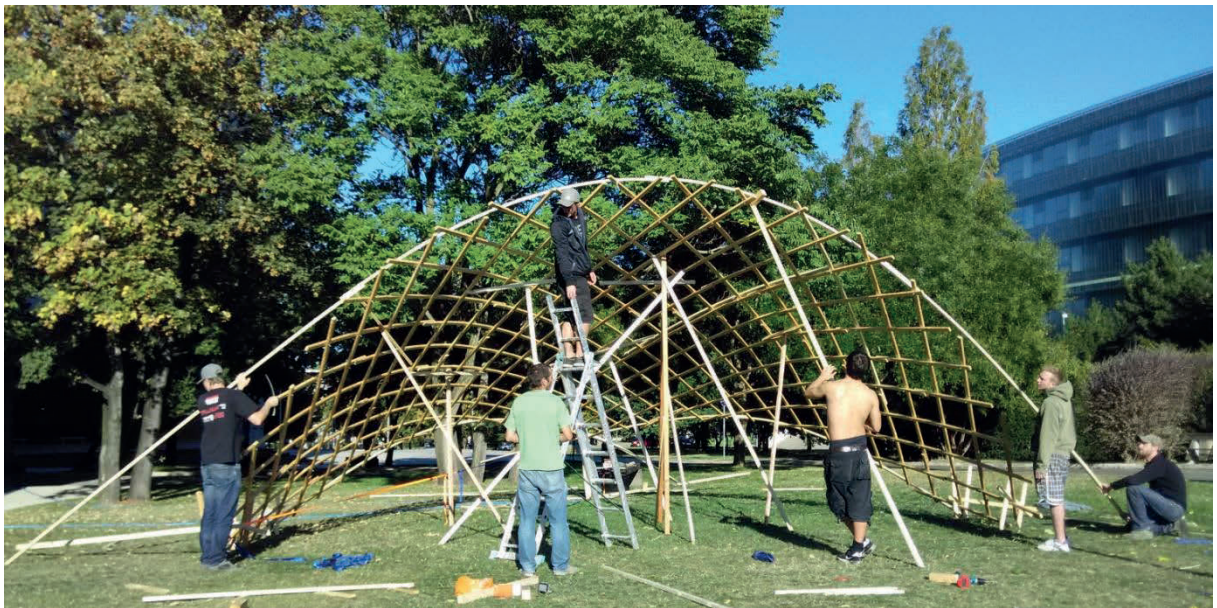
Fig. 6.6 Final shape perimeter tightening [by author 28.9.2015]
