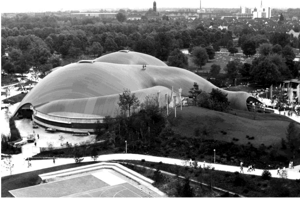
Fig. 2.43 Realization of the Multihall in Mannheim [35]
