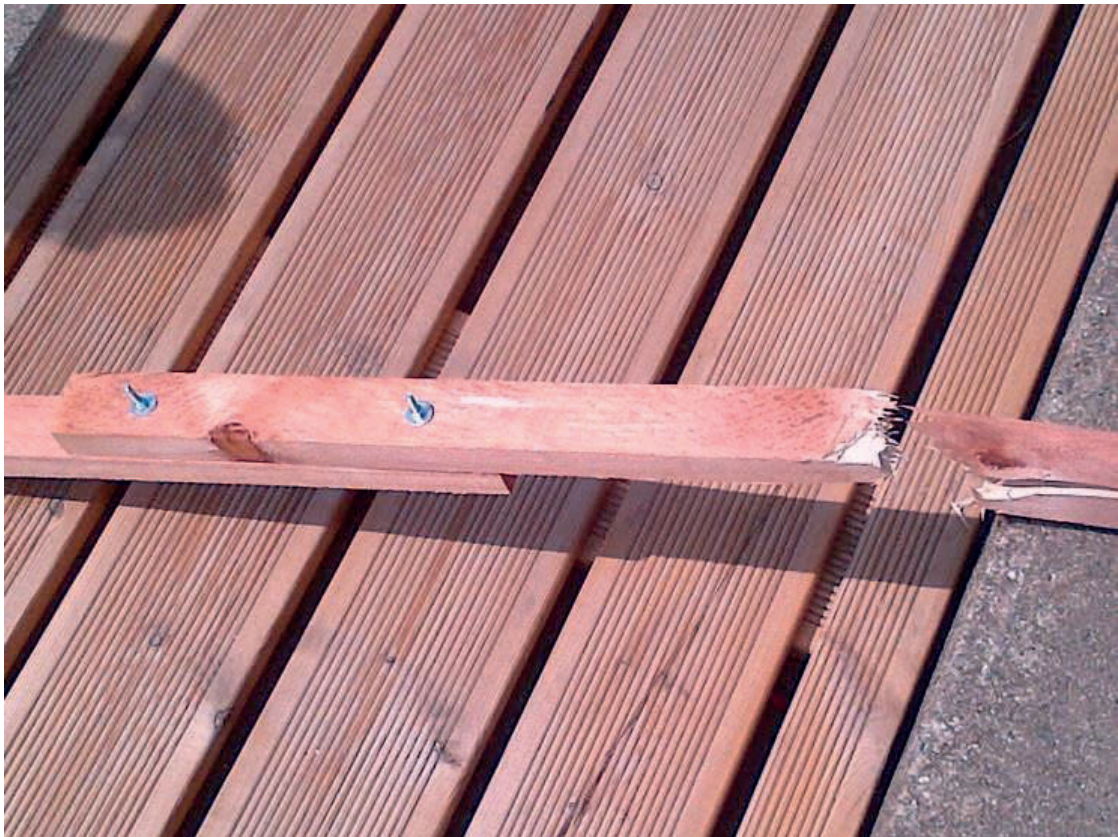
Fig. 4.14 Testing result – breakage near to the longitudinal connection [by author]
