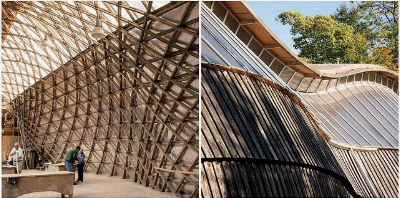
Fig. 2.25 Weald and Downland Museum - completed structure [25]
