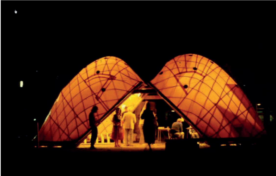
Fig. 2.30 LSRU Grid shell pavilion finished structure at night [27]
