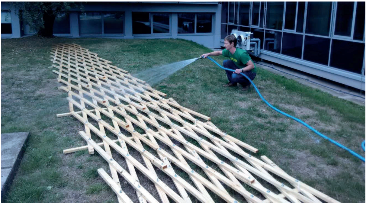
Fig. 3.3 Folded grid, toughen with perpendicular placed laths [by Radomír Vaněk 15.6.2015]
