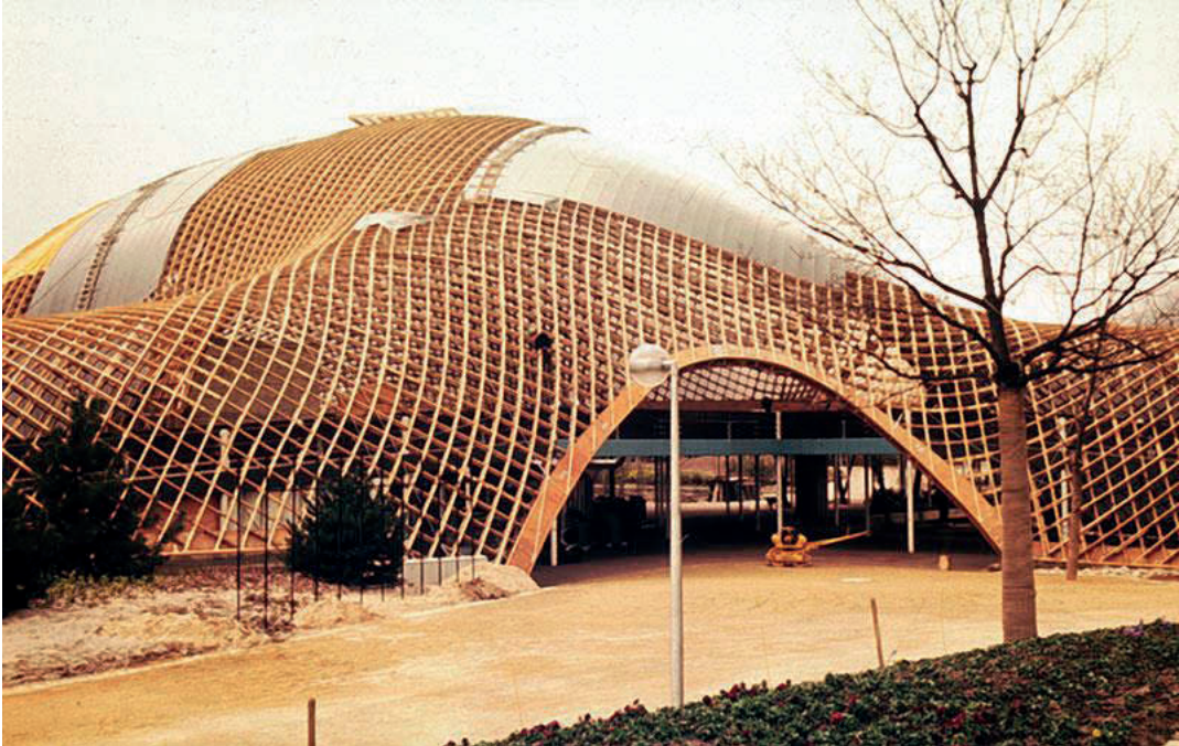
Fig. 2.42 Realization of the Multihall in Mannheim [35]
