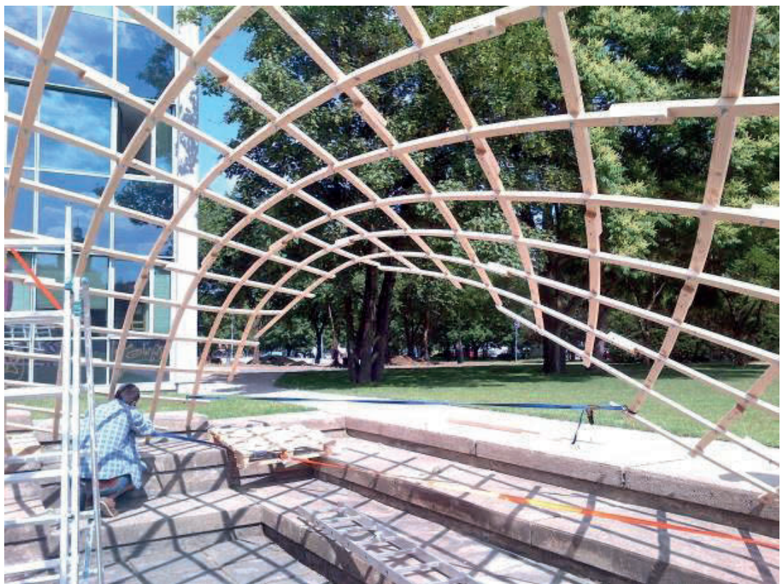
Fig. 3.7 Erecting procedure – inside view [by author 17.6.2015]
