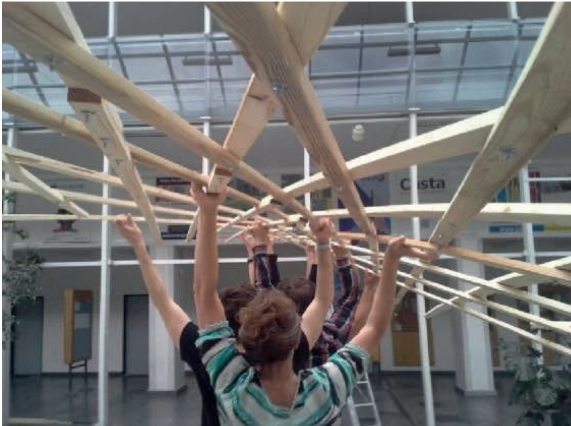
Fig. 3.1 Erection procedure [by author 22.5.2015]
