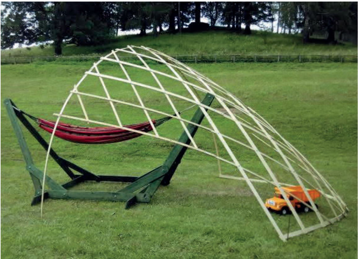
Fig. 3.20 Finished Grid shell cover in the garden [by author]
