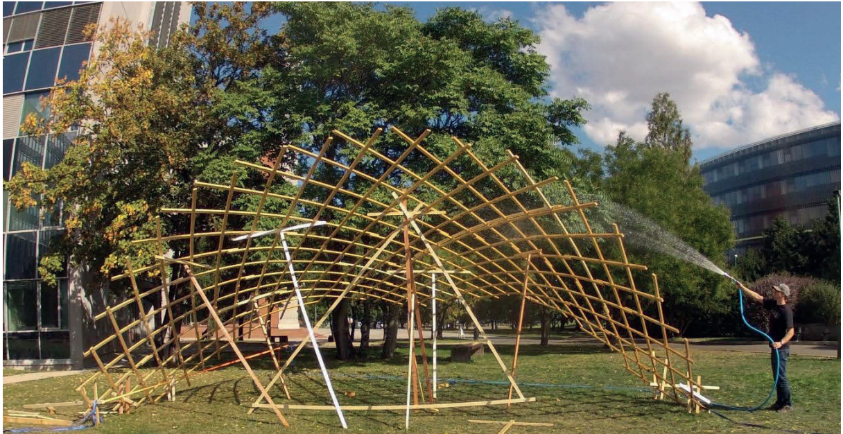
Fig. 6.5 Erecting procedure – Supported and anchored final shape [by author 28.9.2015]
