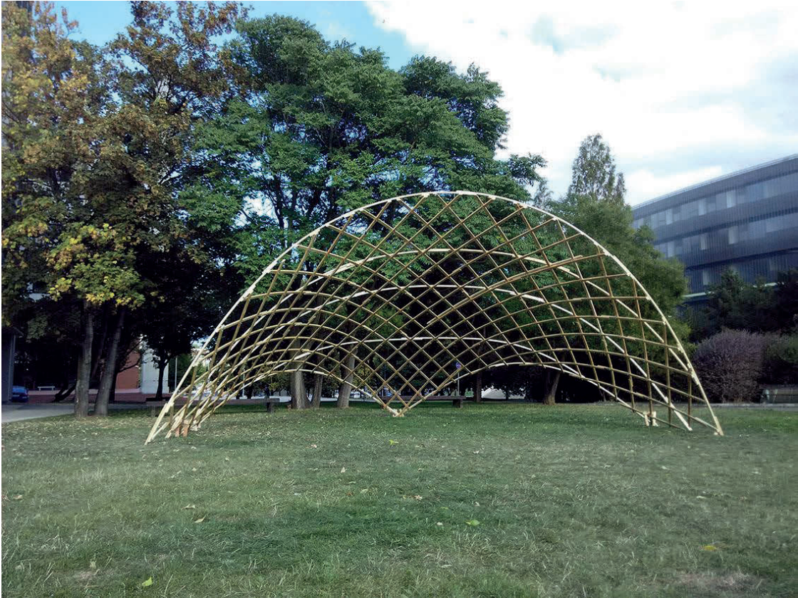
Fig. 8.4 Finished grid shell structure, west view [by author]
