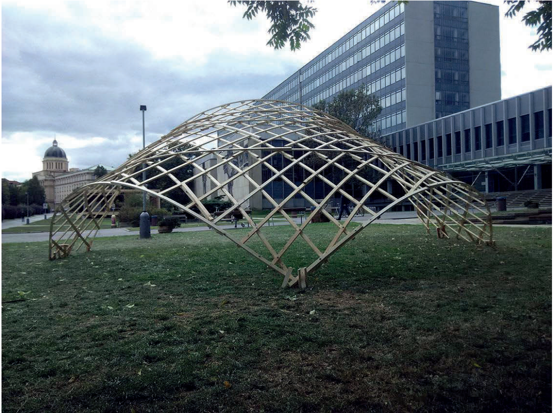
Fig. 8.2 Finished grid shell structure, east view [by author]
