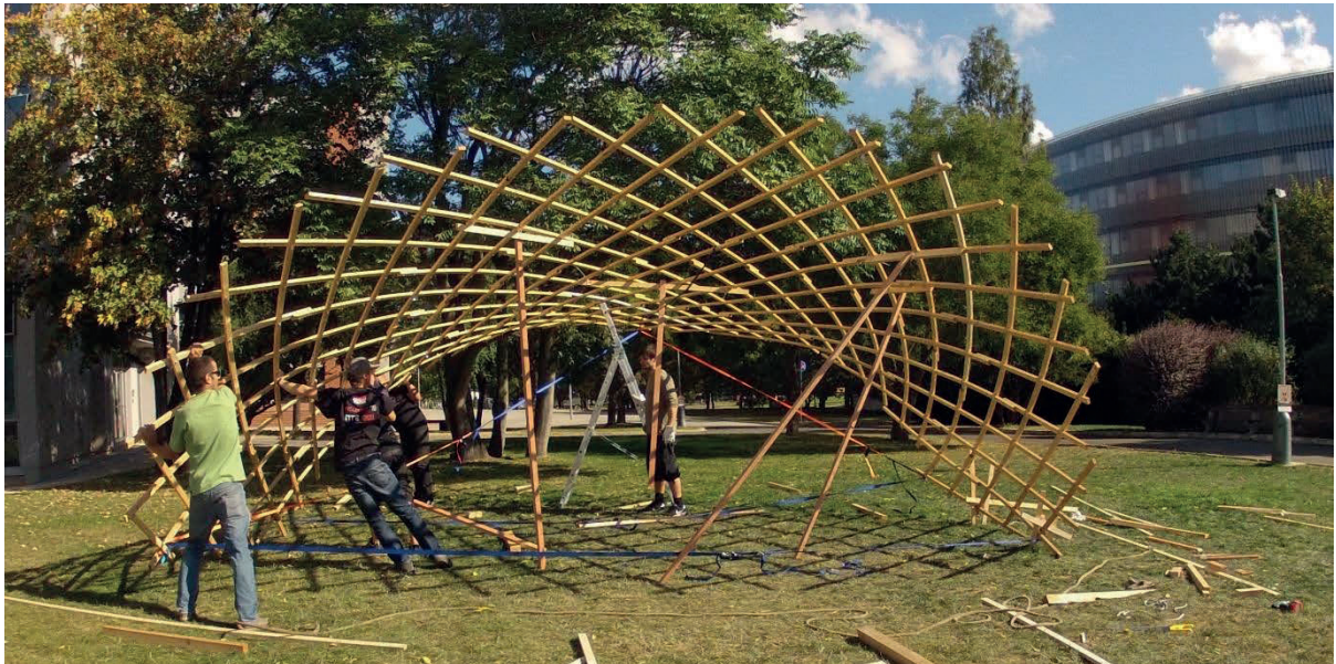
Fig. 6.3 Erecting procedure – lifting up, tightening with belts [by author 28.9.2015]
