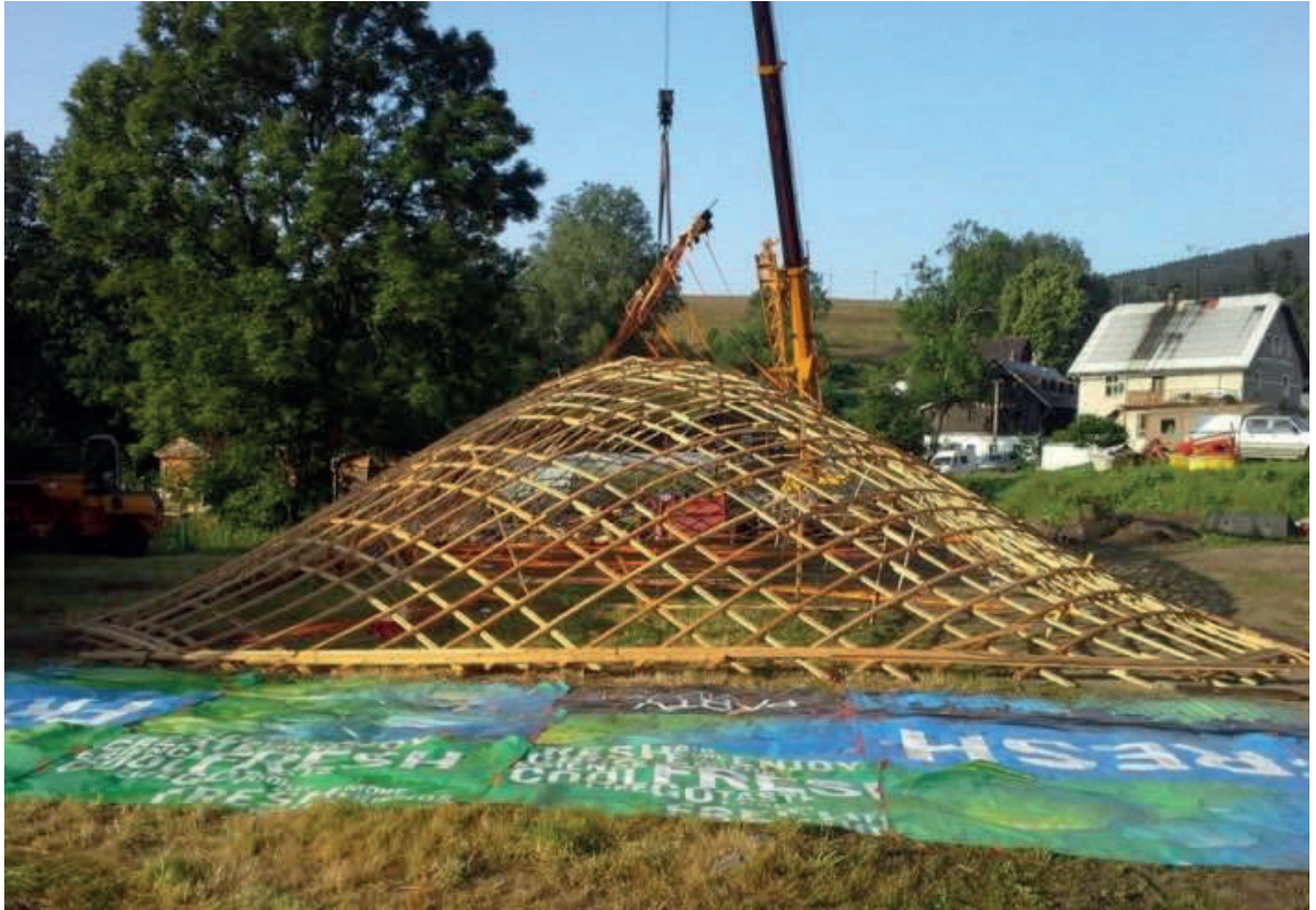
Fig. 3.10 Erected Grid mesh, peripheral fixation [by Radek Podorský 18.7.2015]
