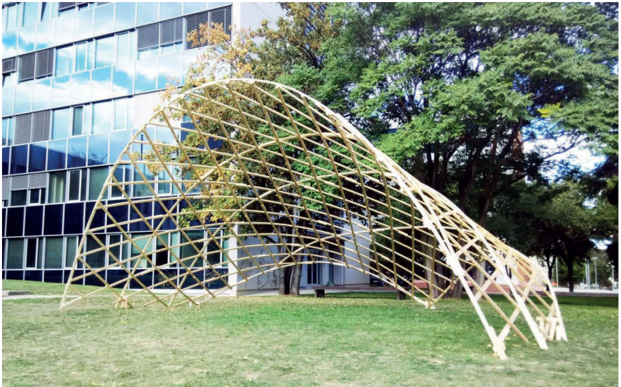
Fig. 8.1 Finished grid shell structure, south-west view [by author]
