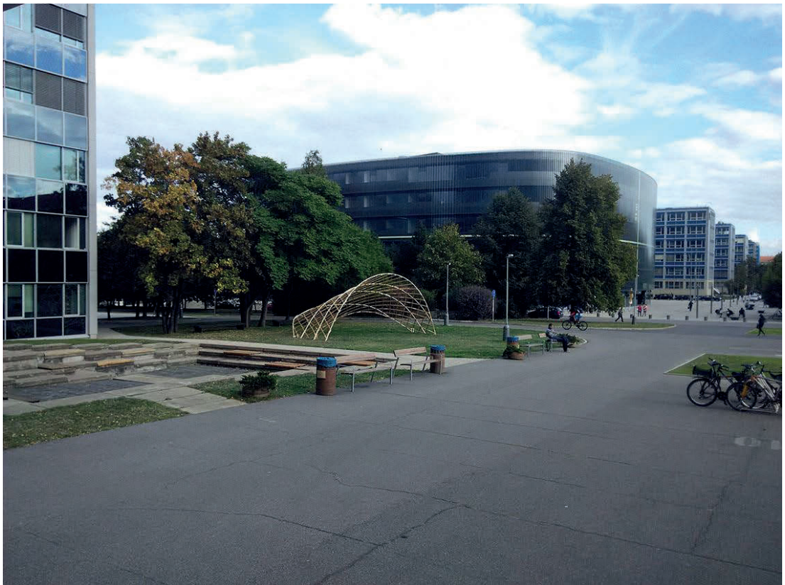
Fig. 8.3 Finished grid shell structure, north-west view [by author]
