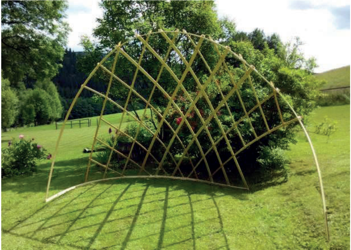
Fig. 3.19 Finished Grid shell cover in the garden [by author]
