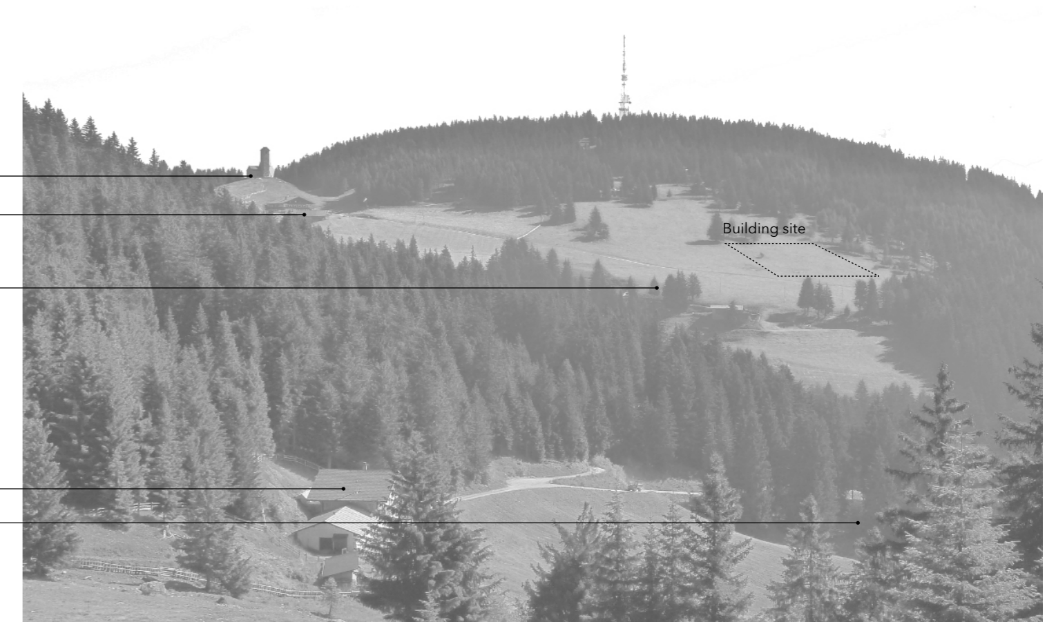
Fig. 24 Facilities and building site on Vigiljoch
