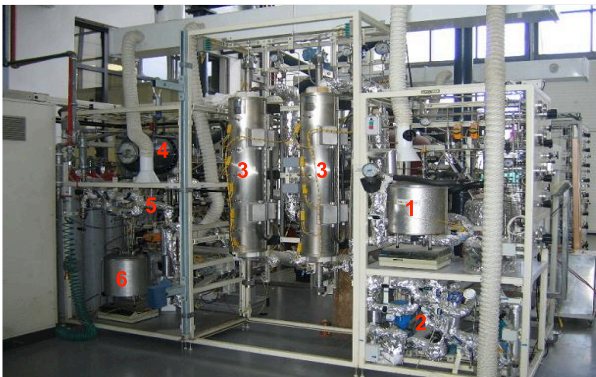
Figure 21: Hydrodesulfurisation pilot plant unit used for hydroprocessing of biowax
