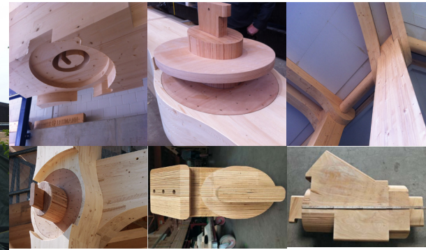
Fig.46: Glulam joints
