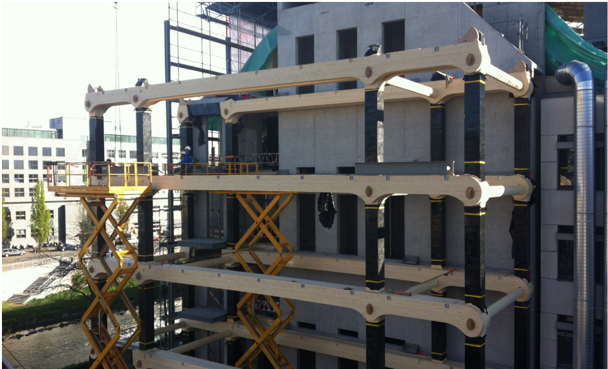
Fig.44: Tamedia building in construction phase
