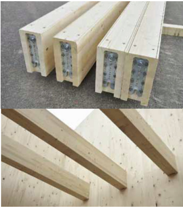
Fig.15: Glulam assembly, joint fastening
