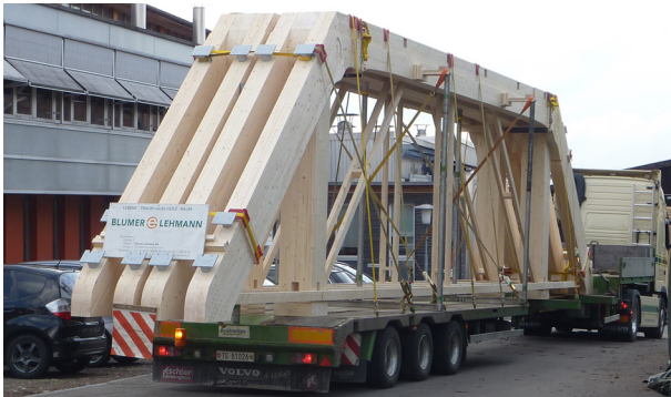
Fig.45: Transportation of elements
