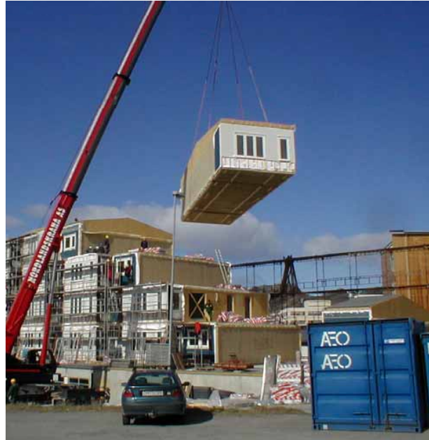
Fig.10: Transporting modules
