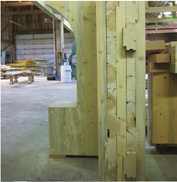
Fig.18: Interlocking CLT principle
