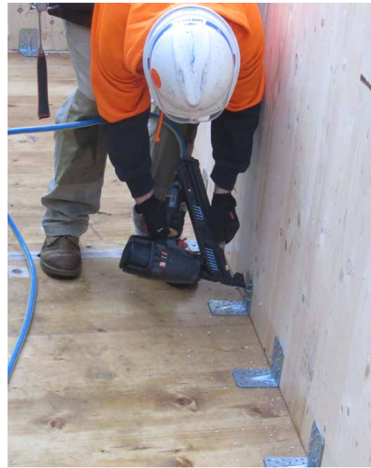
Fig.16: CLT assembly, joint fastening
