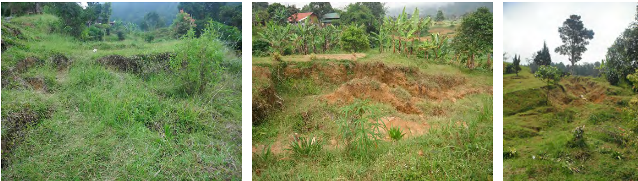
Figure 11: Cracks in the sliding area
