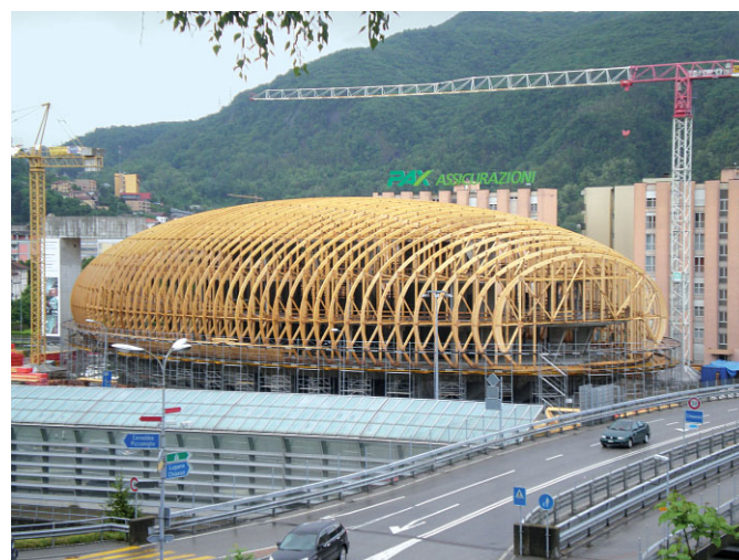
Fig. 1. Formwork for a 93 \times 52 m shell in Chiasso, Switzerland [7] (photo credit: Aurelio Muttoni)
