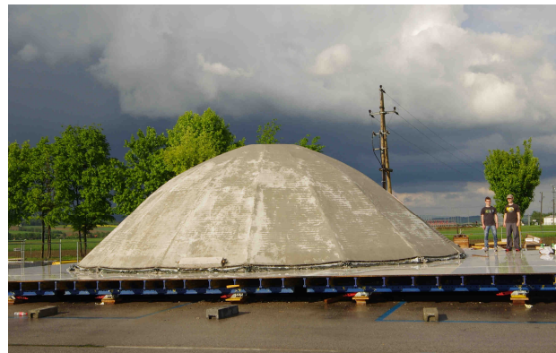
Figure 16: Finished shell structure
