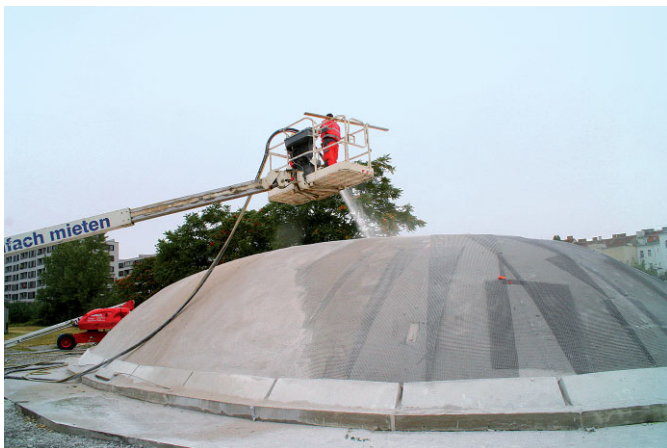
Fig. 24. Applying the layers of sprayed concrete
