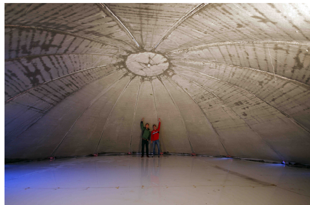
Figure 17: Internal view of the finished shell structure
