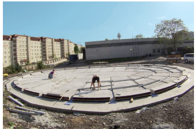
Fig. 17. Installing the lateral displacement protection (steel sections)
