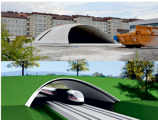
Fig. 25. Application as deer pass (photo credit, visualization: Zechner&Zechner ZT GmbH)
