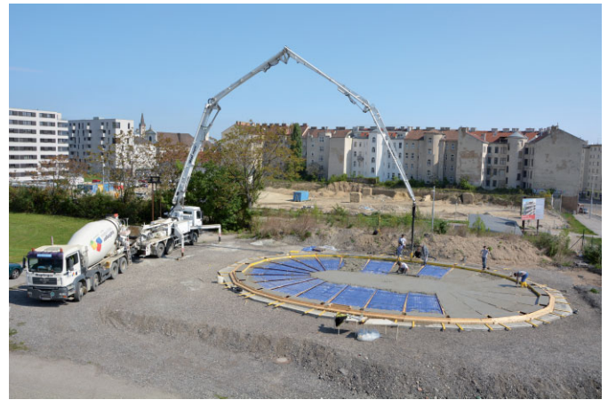
Fig. 16. Casting the flat concrete plate
