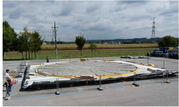
Figure 15: Initially flat concrete plate
