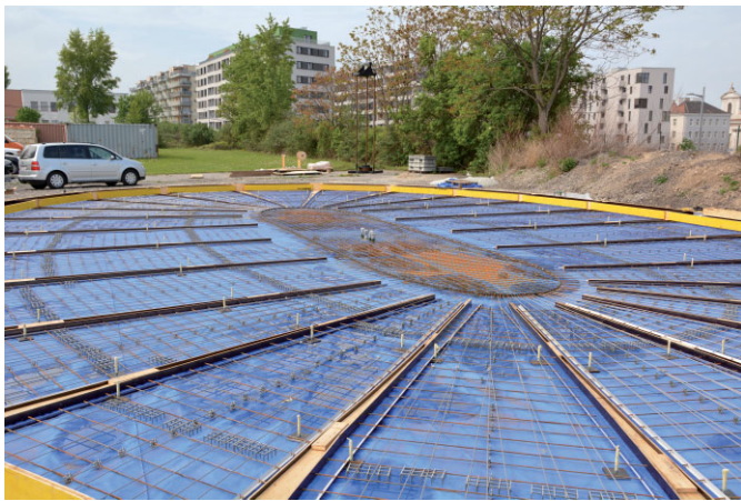
Fig. 15. Formwork with reinforcement already installed
