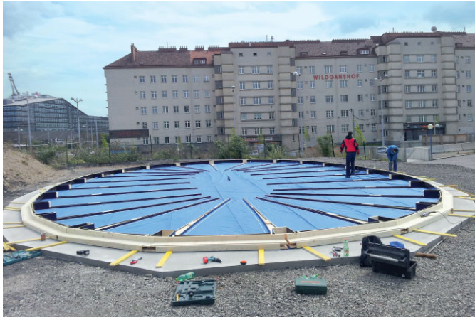
Fig. 14. Fixing the formwork around the circumference and for the wedge-shaped cut-outs
