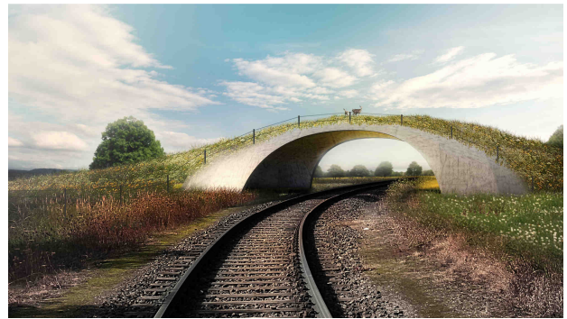
Figure 31: Viaduct for wildlife
