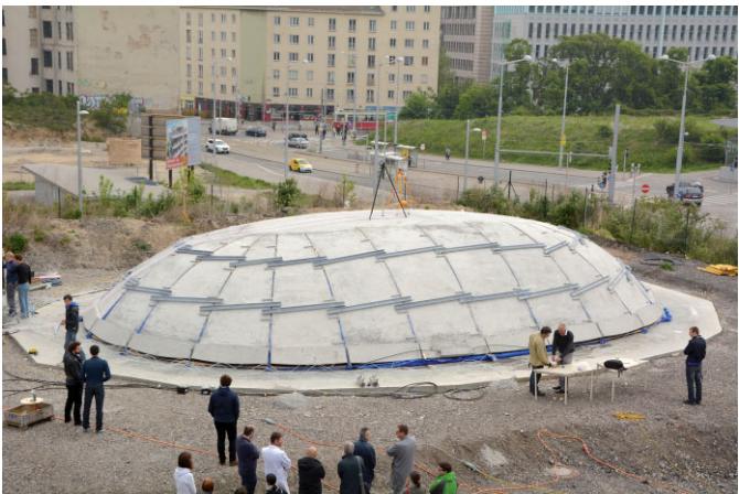
Fig. 18. Transforming a flat plate into a free-form shell
