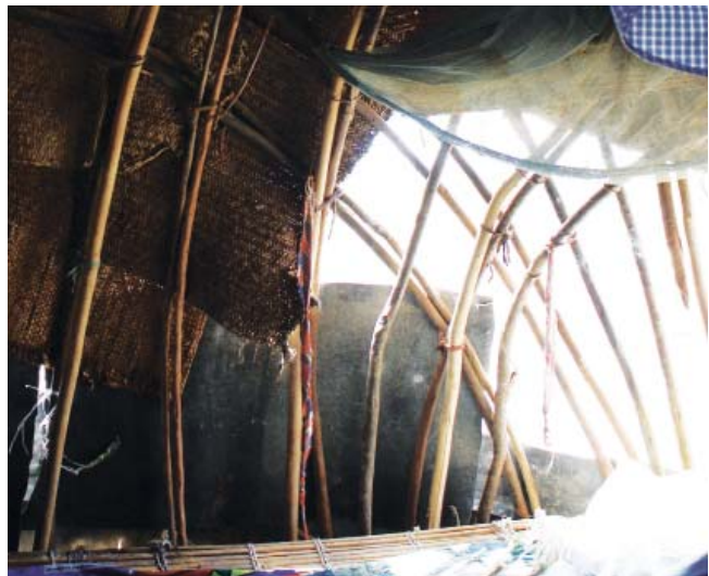
Fig. 277: ventilation opening by the bed at the rear side of daboyta , opened in the morning and closed at night
