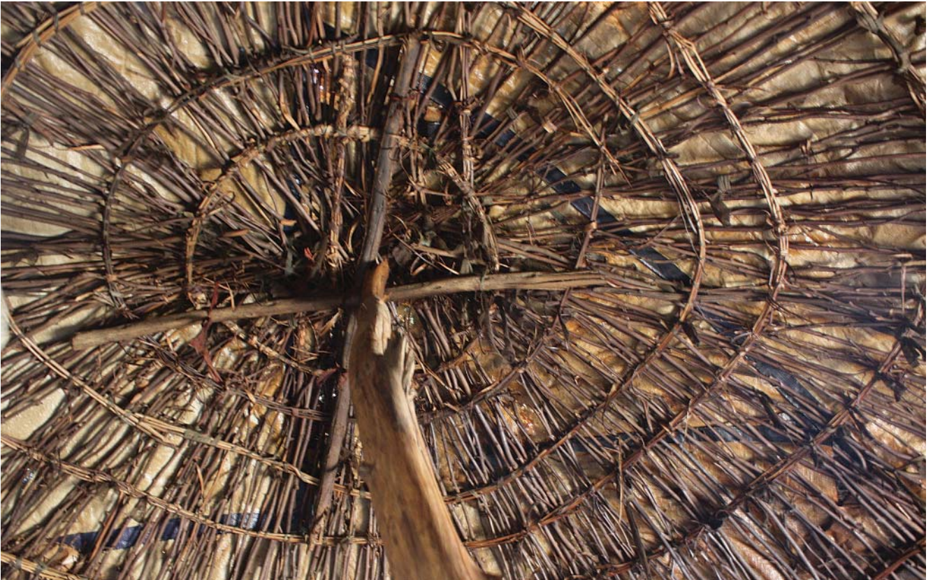
Fig. 299: Gubiyra, Yalo woreda : vertical members are gathered at the crest; the framework is additionally supported at its central point with a single post
