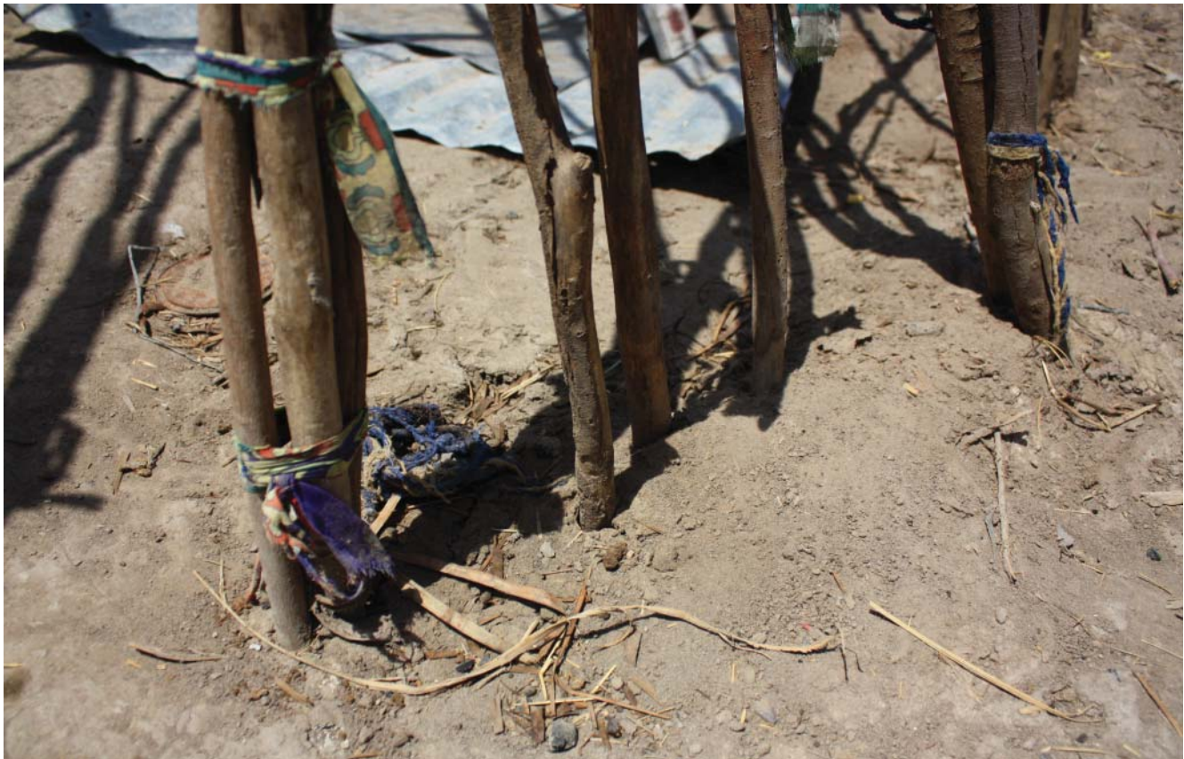
Fig. 259: members of framework of daboyta embedded in the ground
