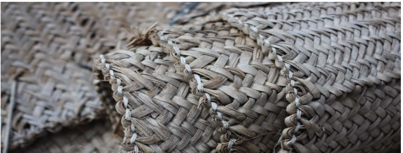
Fig. 250: diagonal braiding of palm mats and fibrous structure of palm leaf allow the water to drain fast from the house cover; the porous structure of material provides both heat and cold insulation, as well as sufficient ventilation
