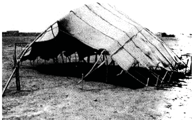
Fig. 200: Hadendowa (Beja), Sudan: house is covered with palm mats; left Prussin et al. 1997:55; right Prussin et al. 1997:5
