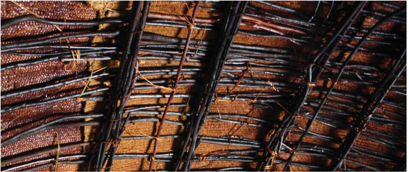
Fig. 232: Logya, Dubti woreda : reinforced rafters of daboyta armature consisting of bundles of acacia roots and branches bound with bark strips
