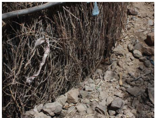
Fig. 309: lower part of a grass hut encased in stones; the house is thatched to the ground
