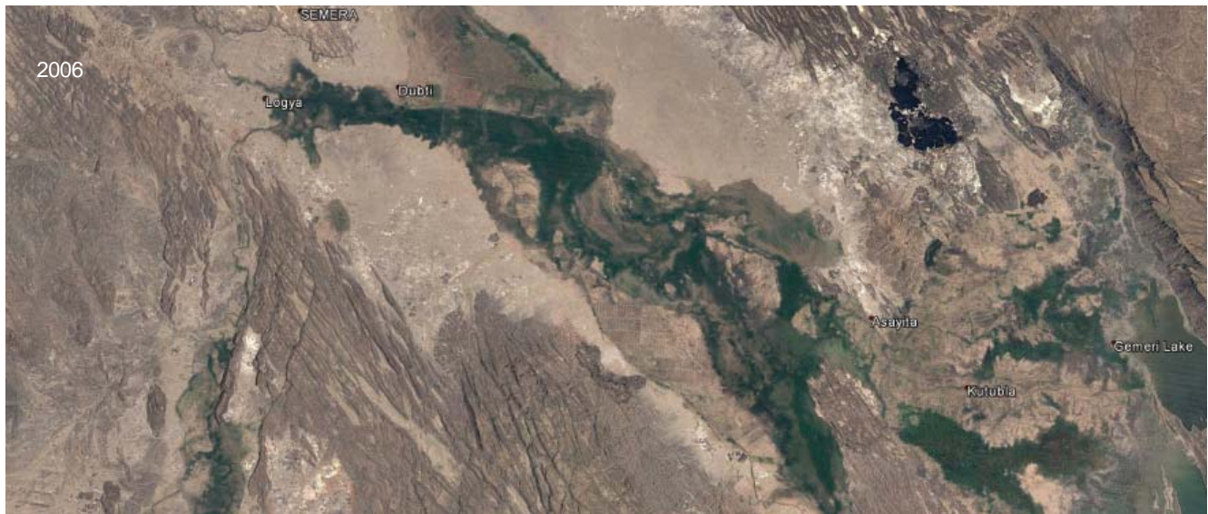
Fig. 158: Dubti and Asayita woreda: 2006-2011 water dam is constructed on the Awash River in Tendaho area; source: Google Earth
