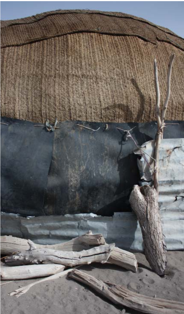
Fig. 266: Logya, Dubti woreda : the cover of daboyta may be complemented with modern materials, or ones found around
