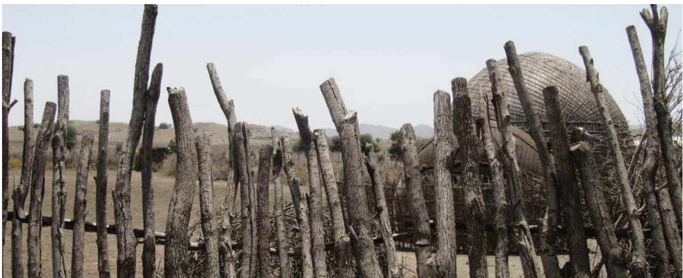
Fig. 81: Alele Subula, Ewa woreda : fence made of branches dug into the ground, forming a palisade
