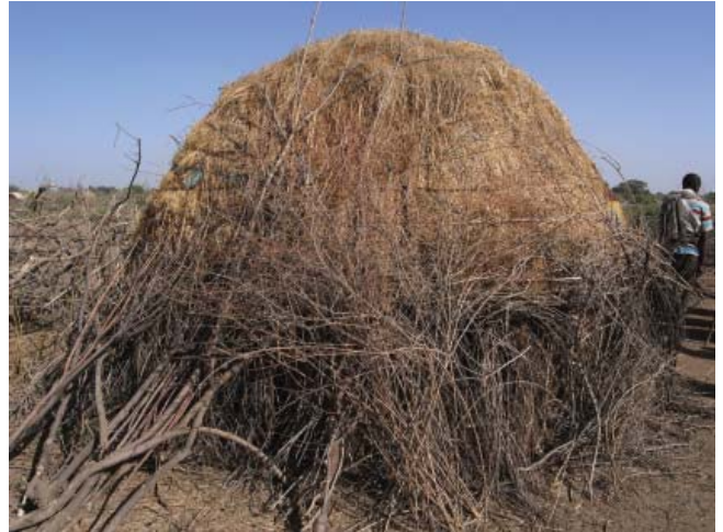
Fig. 307: Ali Adayto, Ewa woreda : lower parts of grass hut are protected by thorn bushes
