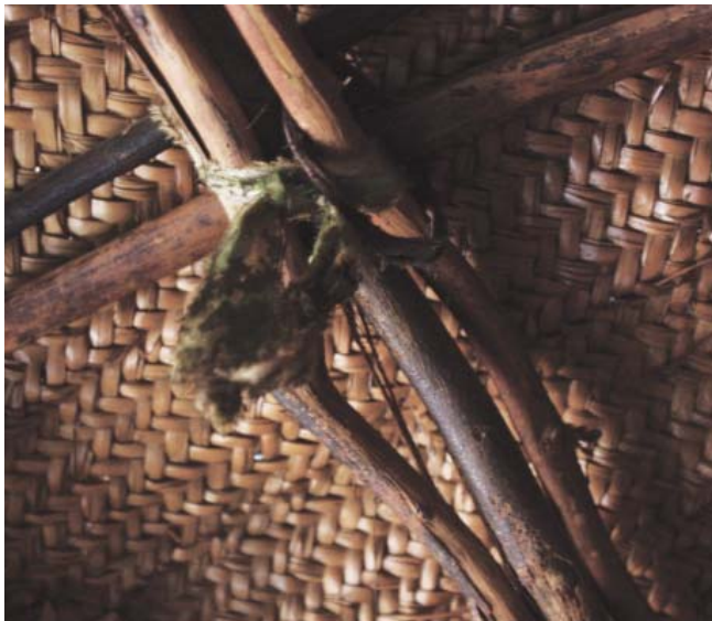
Fig. 261: framework members tied at intersection
