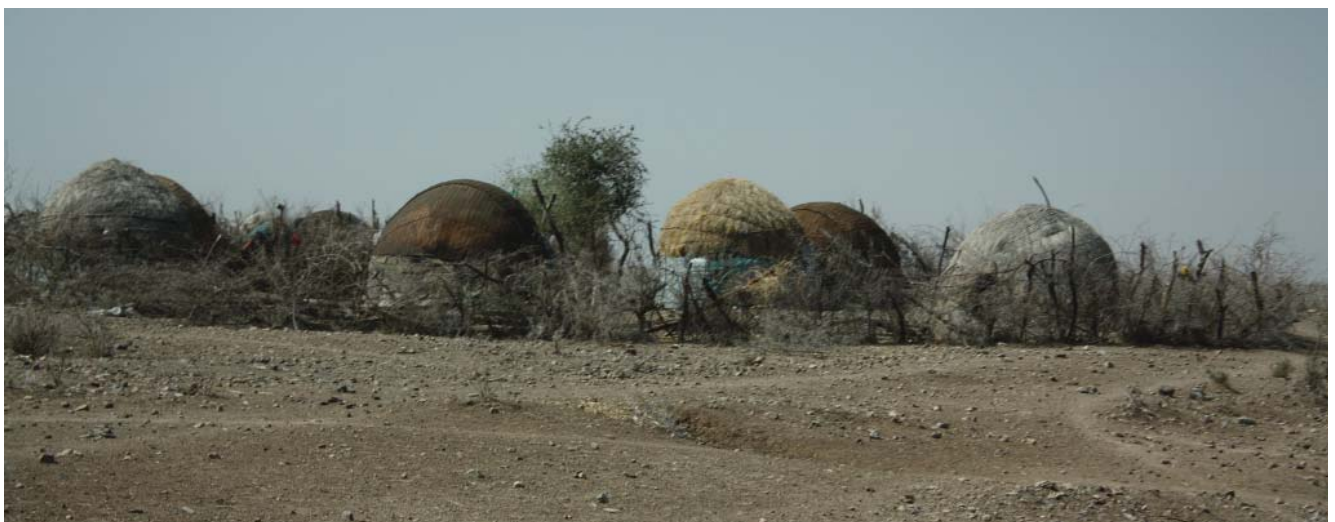
Fig. 62: Chifra woreda: there is no differentiation of built structures within one daala or ganta , which would reflect social hierarchy within community, building effort is a joint undertaking of female community
