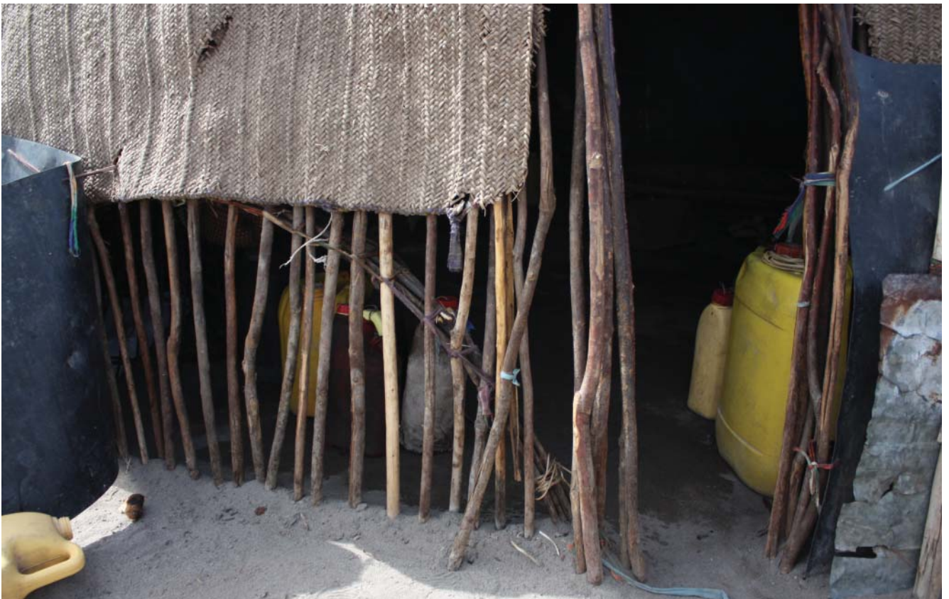
Fig. 275: Logya, Dubti woreda : lower part of daboyta is uncovered so that the air can enter the house; containers with water are placed next to it, so that the water may be kept cool
