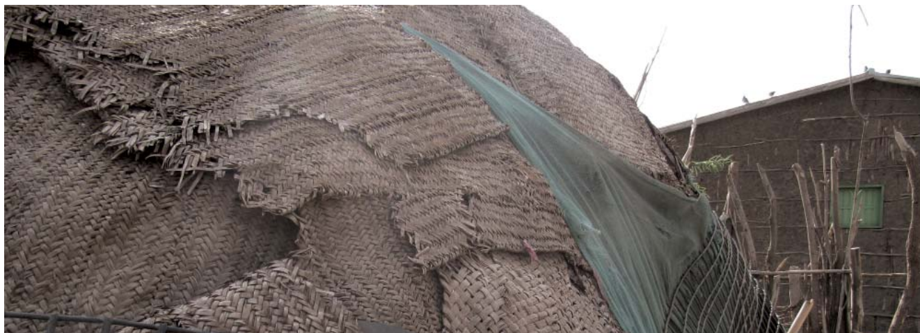
Fig. 268: Logya, Dubti woreda : mats gradually wear out while houses are disassembled and rebuilt many times throughout a year when families migrate between permanent dry season settlements and satellite compounds near the raining pastures
