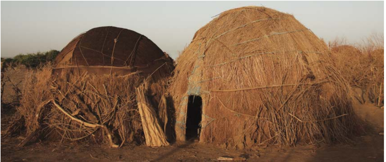
Fig. 215: Ali Adayto, Ewa woreda: typical for this area grass hut adjoining main family house daboyta , which is accessible through the permanent hut
