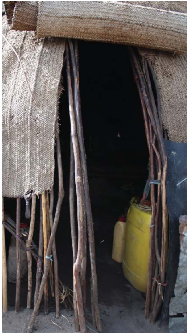
Fig. 328: house entrance closed at night by means of unrolling a mat
