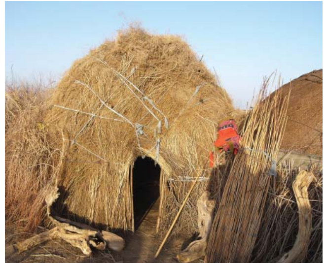
Fig. 303: Ali Adayto, Ewa woreda : thatch wrapped around with ropes
