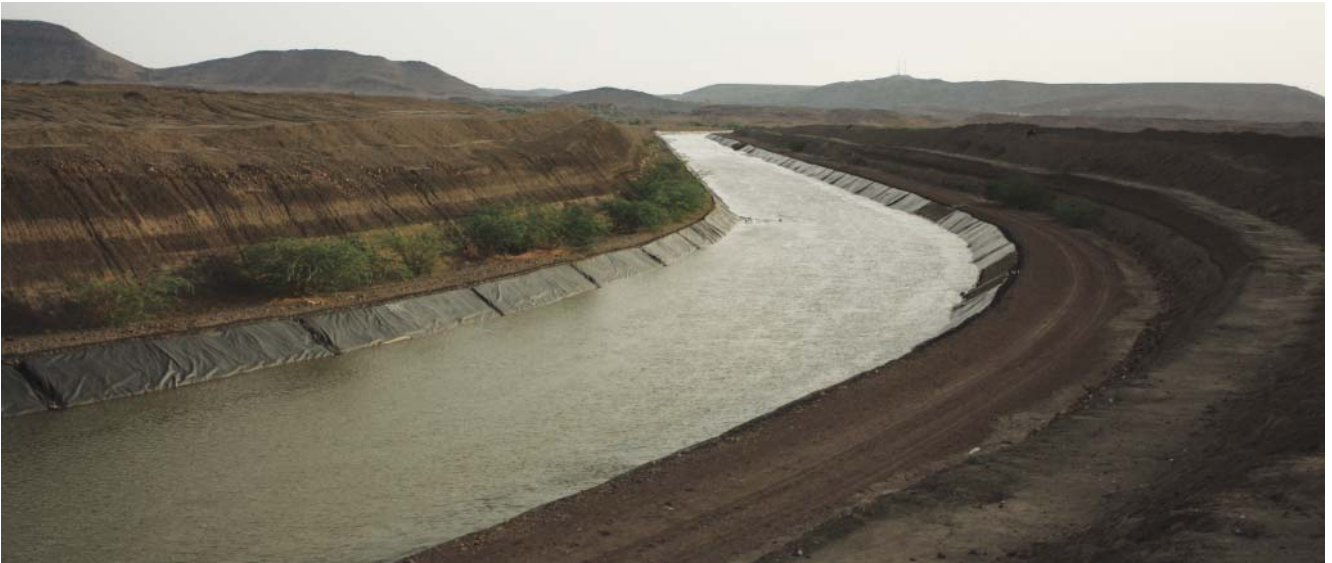
Fig. 161: Dubti woreda : canal channeling water to the sugar cane plant
