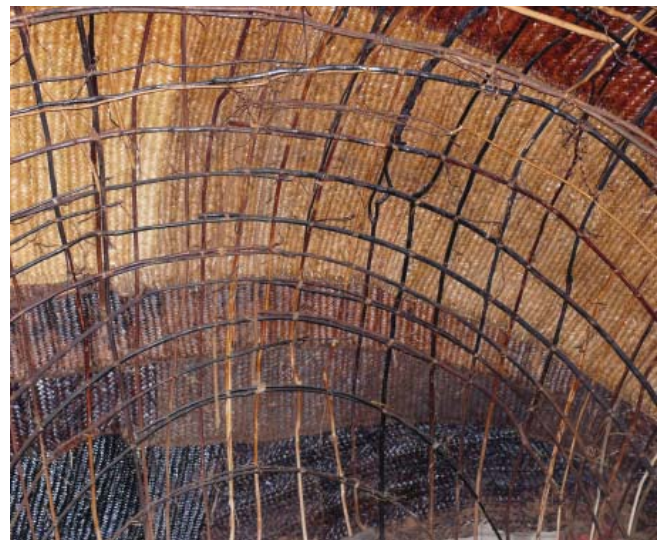
Fig. 234: Ali Adayto, Ewa woreda : armature made of uniform members
