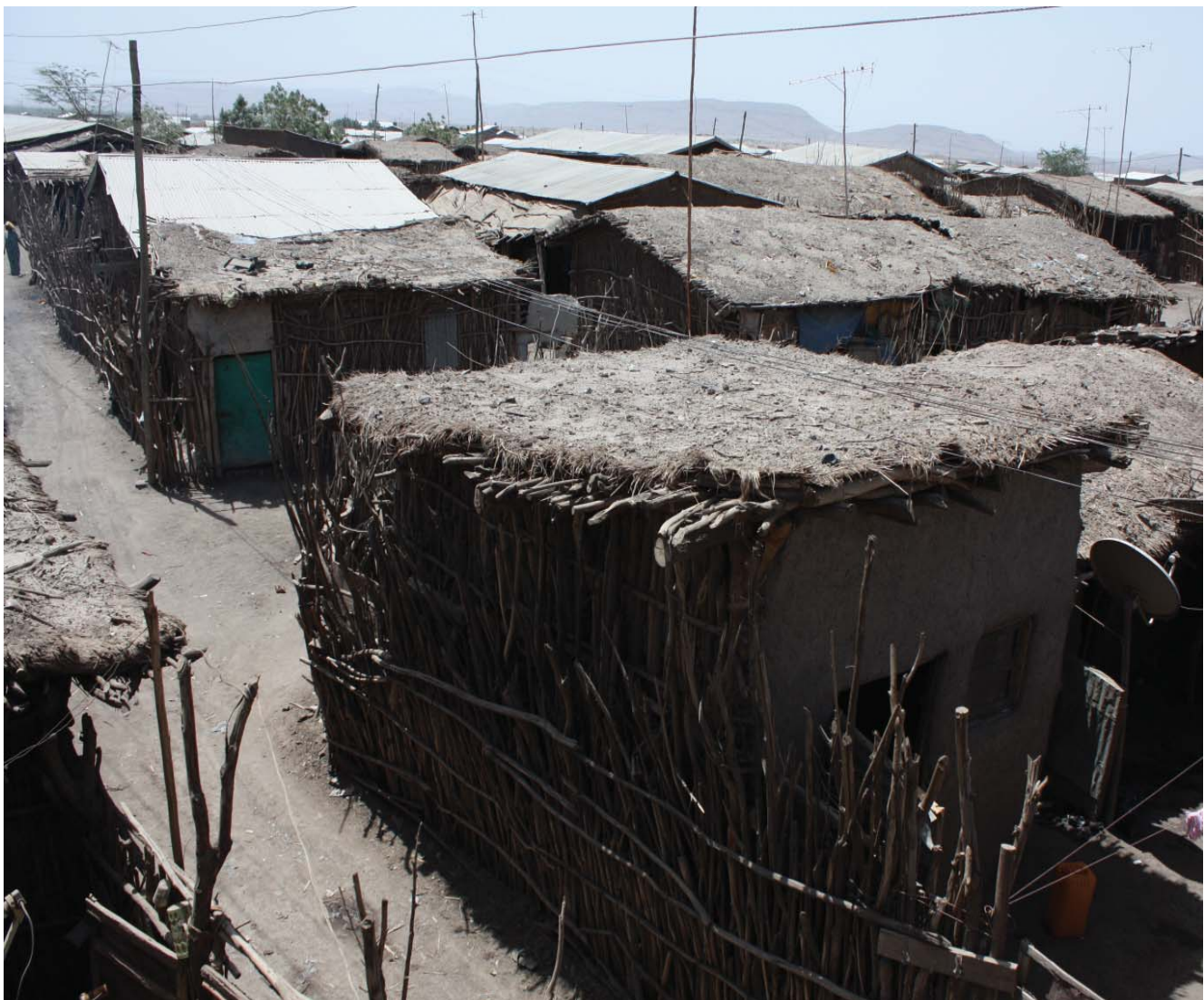
Fig. 155: Logya, Dubti woreda: the growth of urban centres and need to accommodate fast growing number of people led to expansion of ch'qa building technique, which utilizes wood as main building resource and which highly contributed to the acceleration of deforestation
