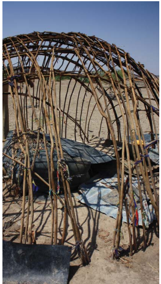
Fig. 242: Logya, Dubti woreda : entrance built in the armature
