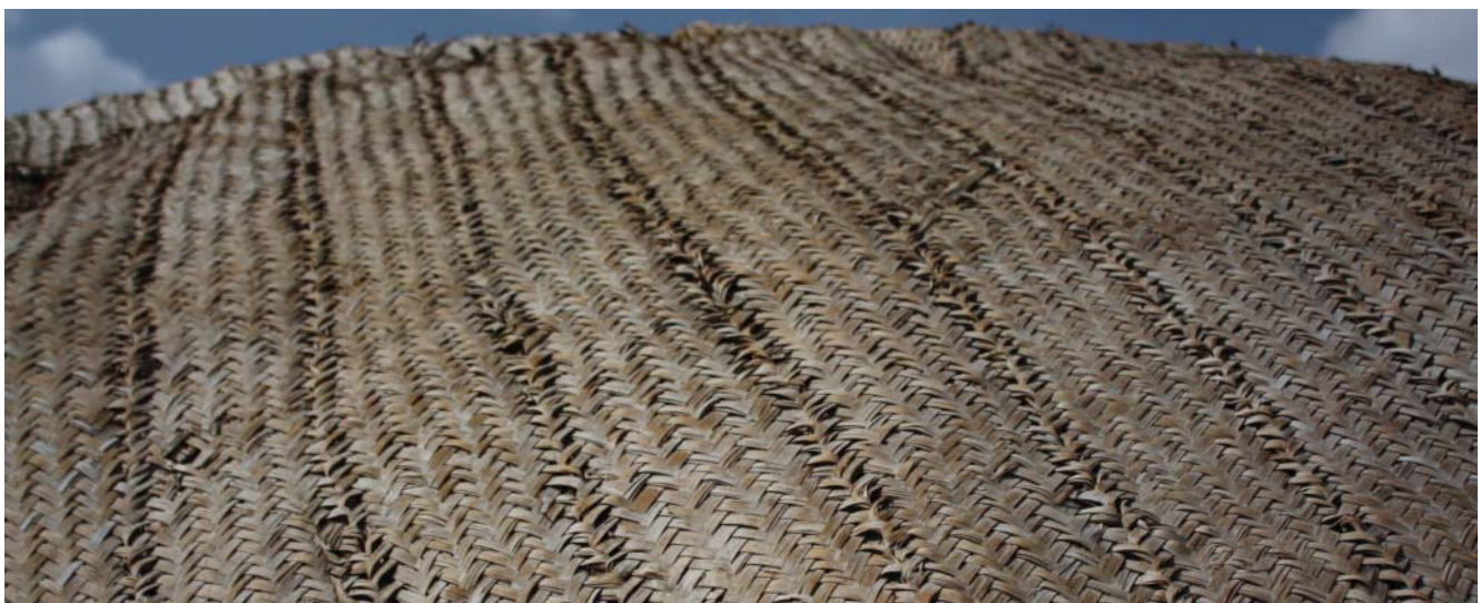
Fig. 252: palm mat is made of strips of woven palm leaves, which are sewn together; the number of strips depends on the desired length of the mat
