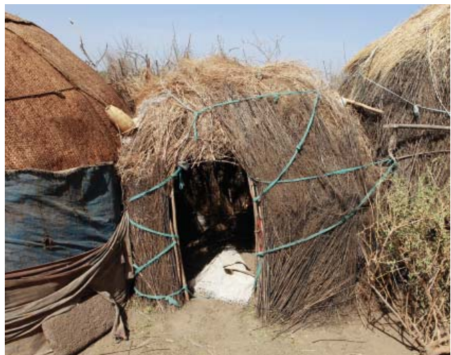
Fig. 214: Ali Adayto, Ewa woreda : thatched middle hut joining daboyta with grass hut , through which both are accessible
