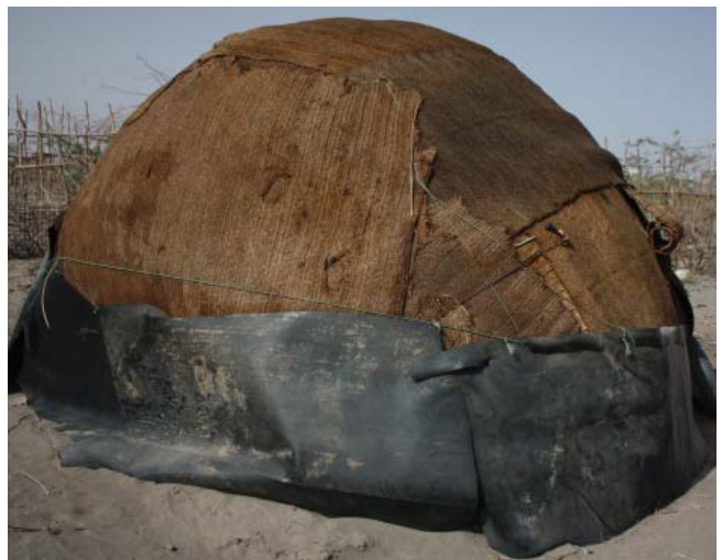
Fig. 267: Logya, Dubti woreda : mats gradually lose their flexibility and water tightness due to the sun radiation
