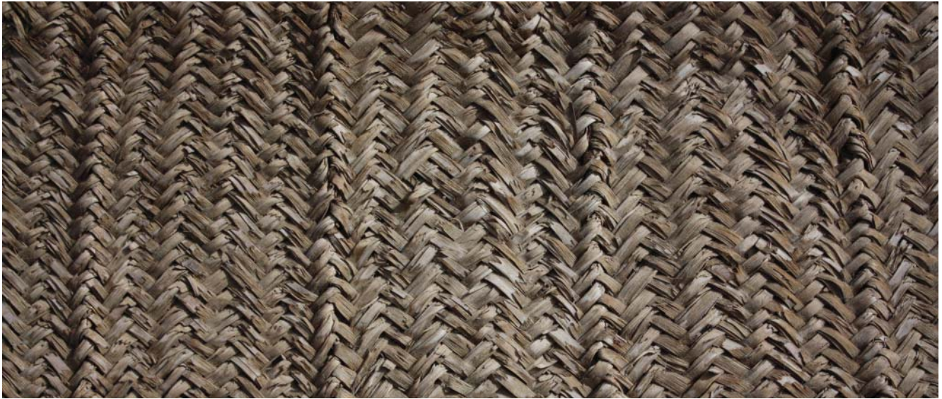
Fig. 269: insulating qualities of palm mats allow to keep the inside of the tent relatively warm during cold nights and cool during the heat of the day
