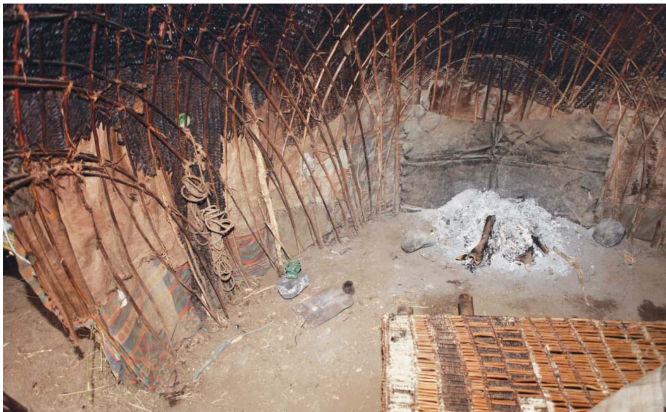
Fig. 357: Ali Adayto, Ewa woreda : a hearth inside daboyta : smoke seeps through the pores of the roof; a proper ventilation is difficult when all mats are closed, because the entrance to daboyta leads through the grass hut , there is no direct outlet to the outside but through the mats
