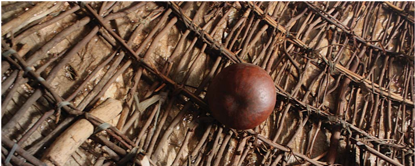
Fig. 301: dense arrangement of vertical and horizontal members, which are joined at the intersections, gives the framework desired stability
