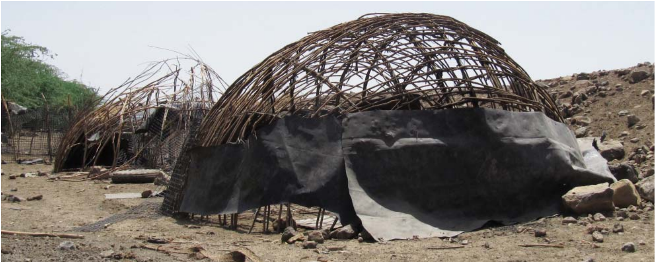
Fig. 241: Dubti woreda : complete armature of abandoned daboyta ; in the background: some of the members have been removed and taken to the permanent settlement, where they will be used to construct a smaller daboyta
