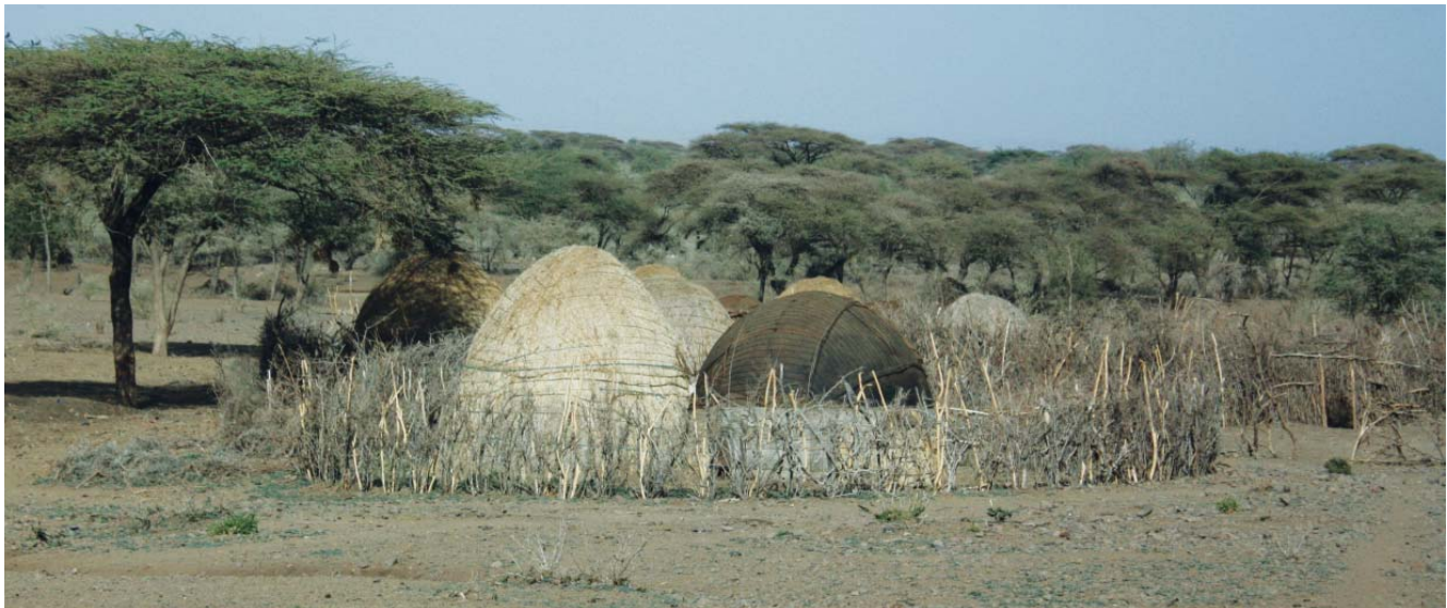
Fig. 51: Ewa woreda: compound of an extended family comprising permanent grass huts (front left) and mobile mat daboytas (front right)
