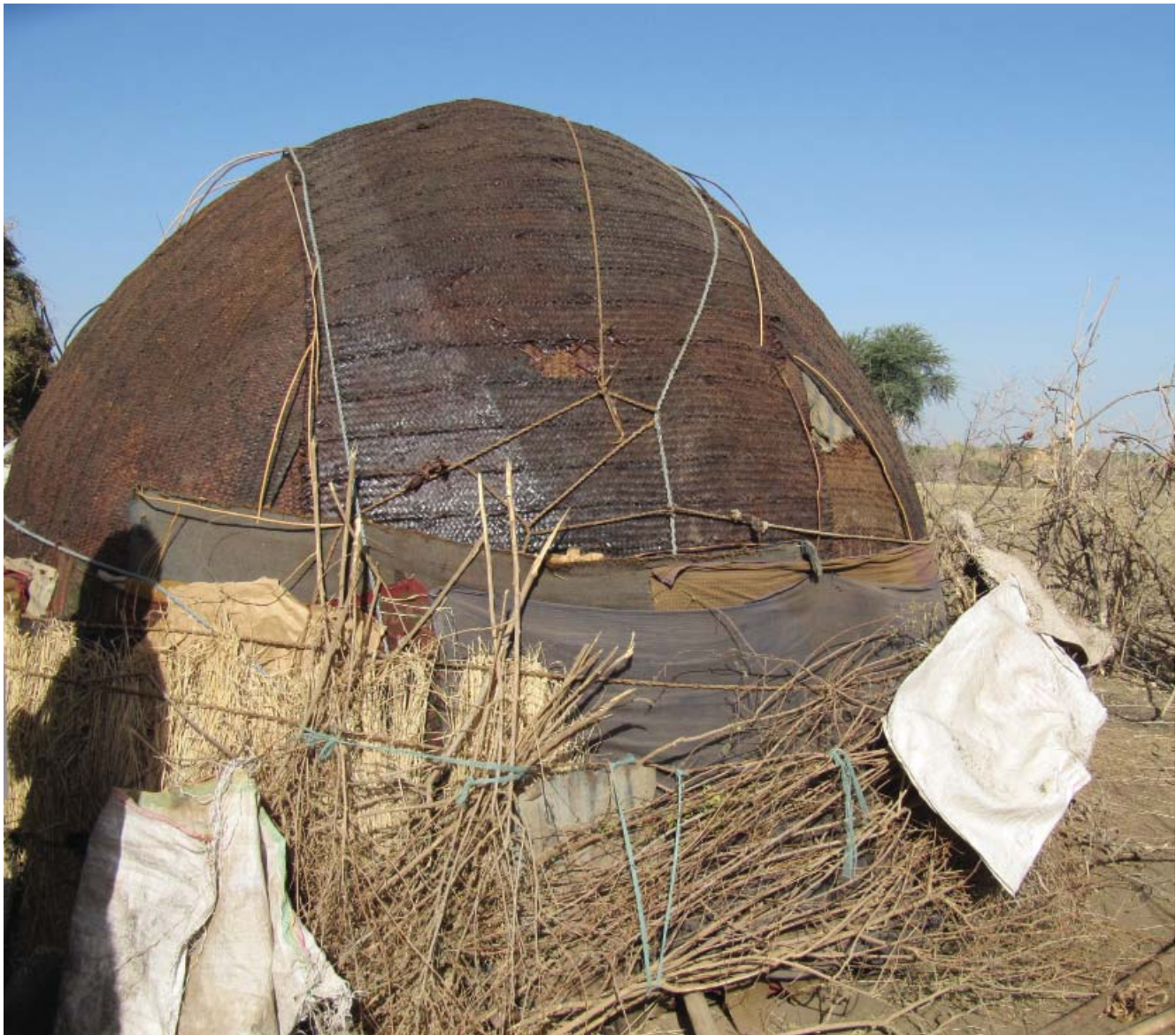
Fig. 235: Ali Adayto, Ewa woreda: daboyta considerably extended in height, such form enhances its stability in the windy area
