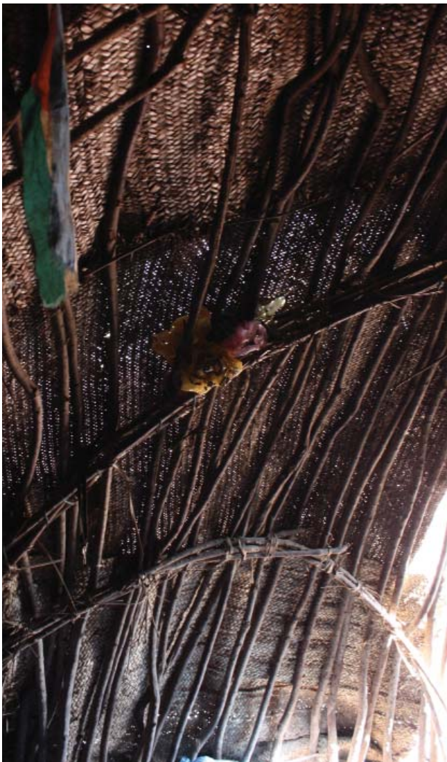
Fig. 244: Semera, Dubti woreda : reinforcement arches installed at the bottom of an armature on both sides of an entrance replacing main construction arch that would run here otherwise if there was no opening
