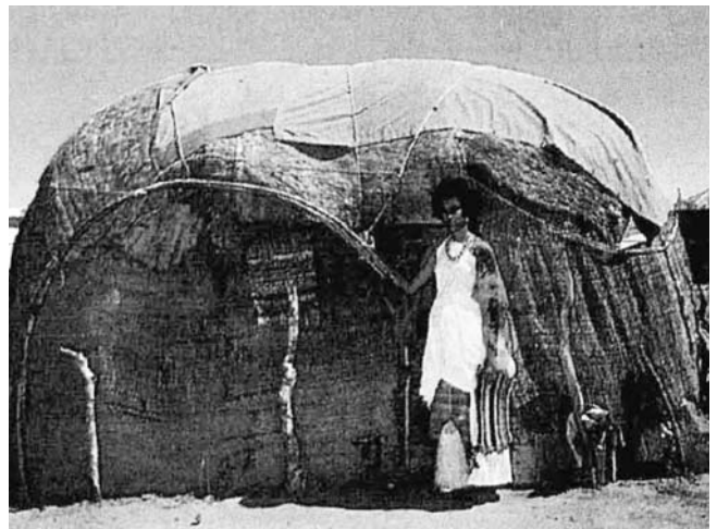
Fig. 208: Somali, Ethiopia: armature covered with mats made of a mixture of sisal and acacia fibres; Oliver 1997:2028
