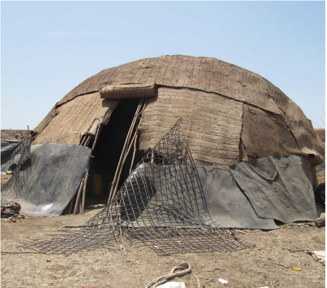
Fig. 211: Dubti: a regular daboyta - round house covered with palm mats; at the bottom complemented with plastic foil
