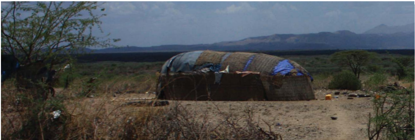
Fig. 209: Amibara woreda : elongated house covered with reed mats complemented with waterproof foils
