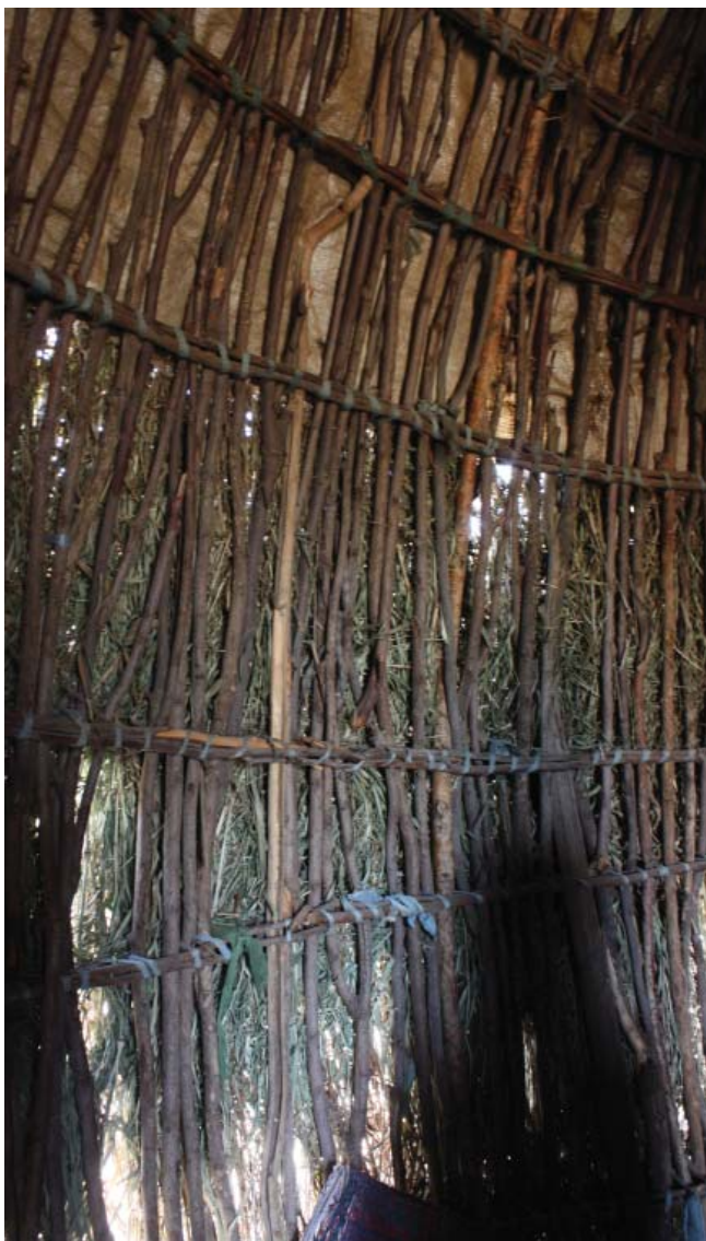
Fig. 298: Gubiya, Yalo woreda : regular framework of vertical members stabilized with horizontal bracing
