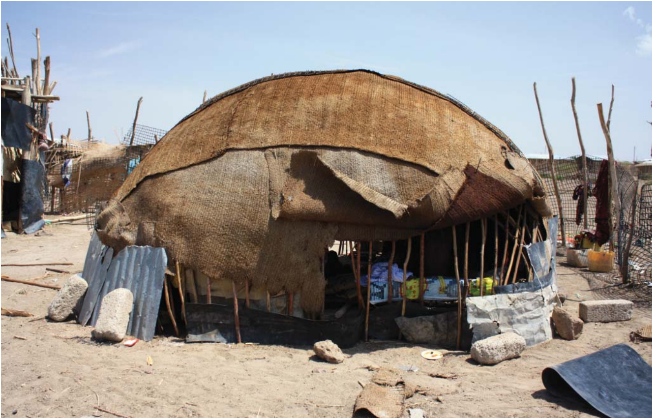
Fig. 274: Logya, Dubti woreda : lower side mats are rolled up to allow air movement through daboyta
