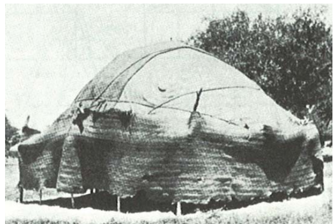
Fig. 202: Touareg central-western Sahara: armature dwelling covered with palm mats; Denyer 1978:104
