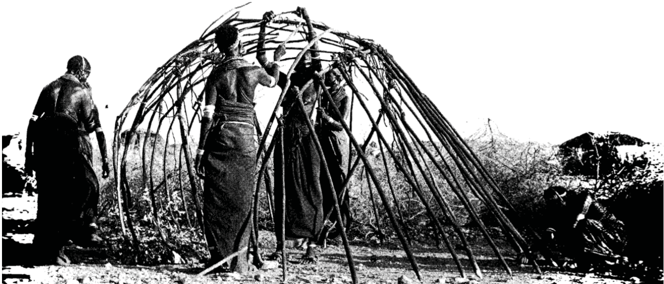
Fig. 198: Rendile, Kenya: armature dwelling; house is covered with hand-woven grass mats; Prussin 1997:157
