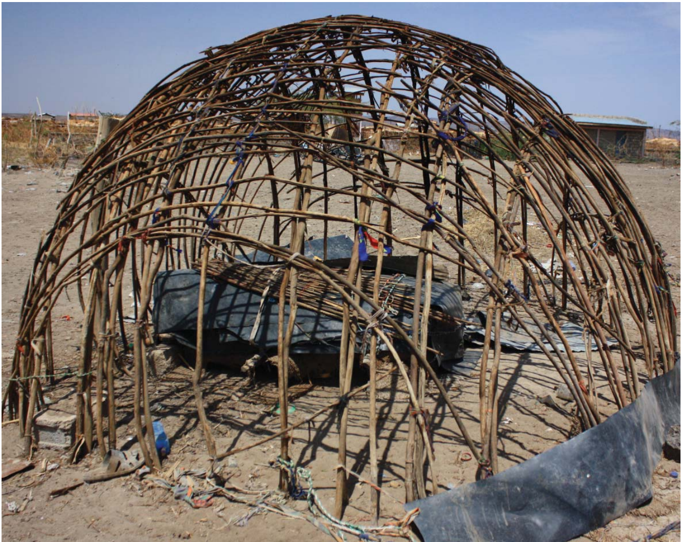
Fig. 221: Logya, Dubti woreda : armature of abandoned daboyta ; bed frame and some mats are stored under foil, protected from rain and sun
