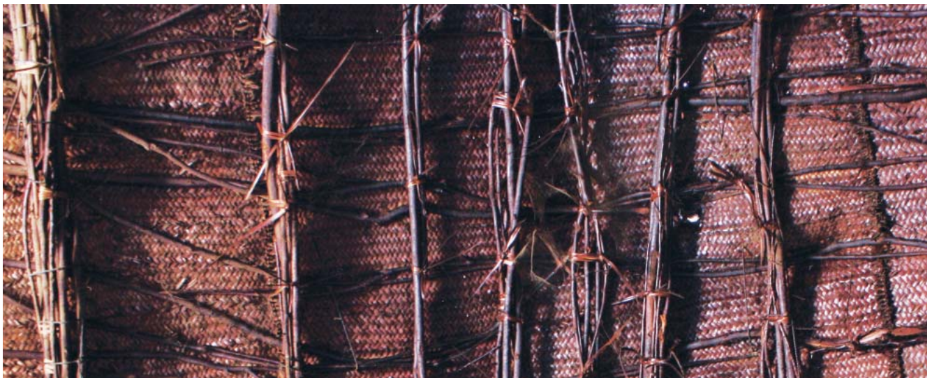
Fig. 254: natural bark, sisal ropes or thongs are used for tying elements of armature together; thorns and ropes are used to tie mats to framework
