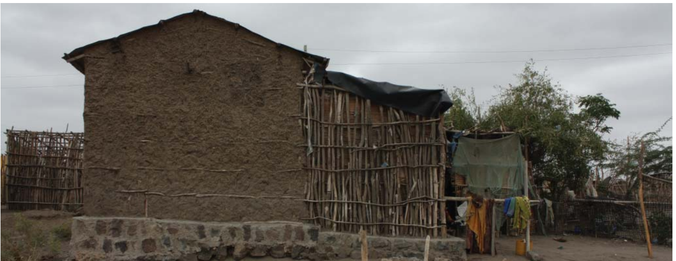
Fig. 220: Logya, Dubti woreda : a house of an settled Afar built in ch'qa technique: palisade of relatively straight woods is embedded in the ground and plastered in three layers with mud mixed with straw; the stone „foundation“ is built around the house, but it does not bear any loads
