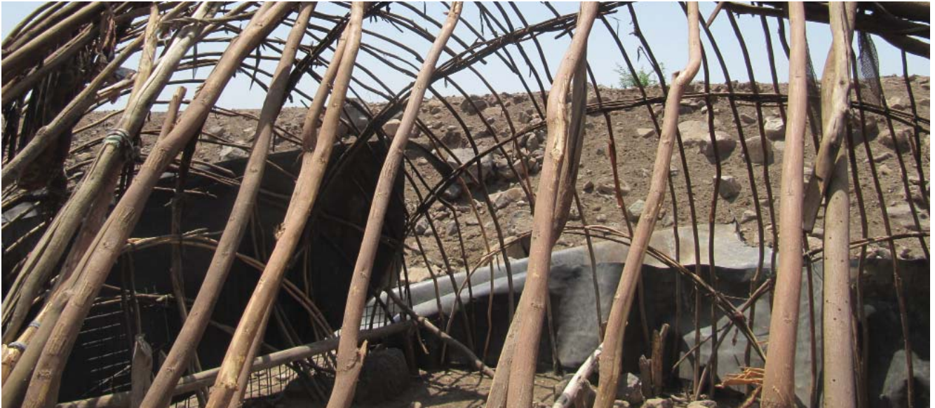
Fig. 249: Dubti woreda , acacia members of an armature of a daboyta left behind in the main dry season compound; shorter pieces are tied together in bundles to form longer members needed to cover the longitudinal or transverse span of a house
