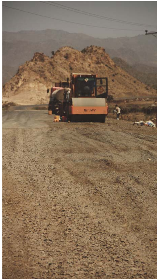
Fig. 09: Afdera-Mekele road under construction (Chinese contractors)
