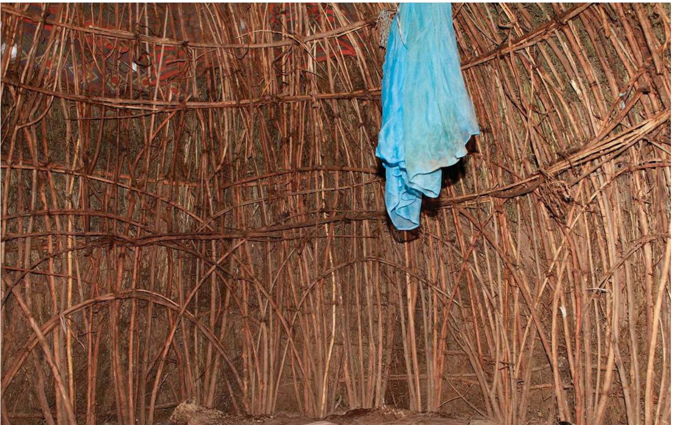
Fig. 300: Ali Adayto, Ewa woreda : grass huts of bigger size may have additional bracing introduced in form of arches encircling the bottom part of a framework; the horizontal bracing starts at the height of about 60cm above the floor - just above the bracing of arches
