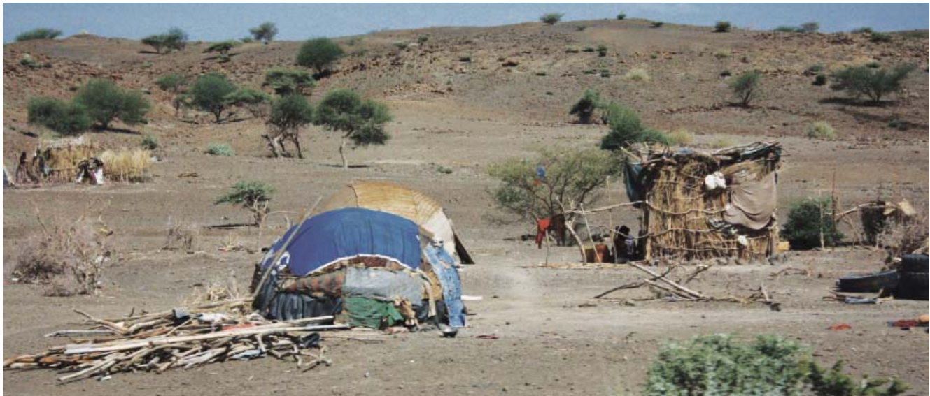
Fig. 255: Mile woreda : the use of modern cover materials complements the repertoire of natural ones
