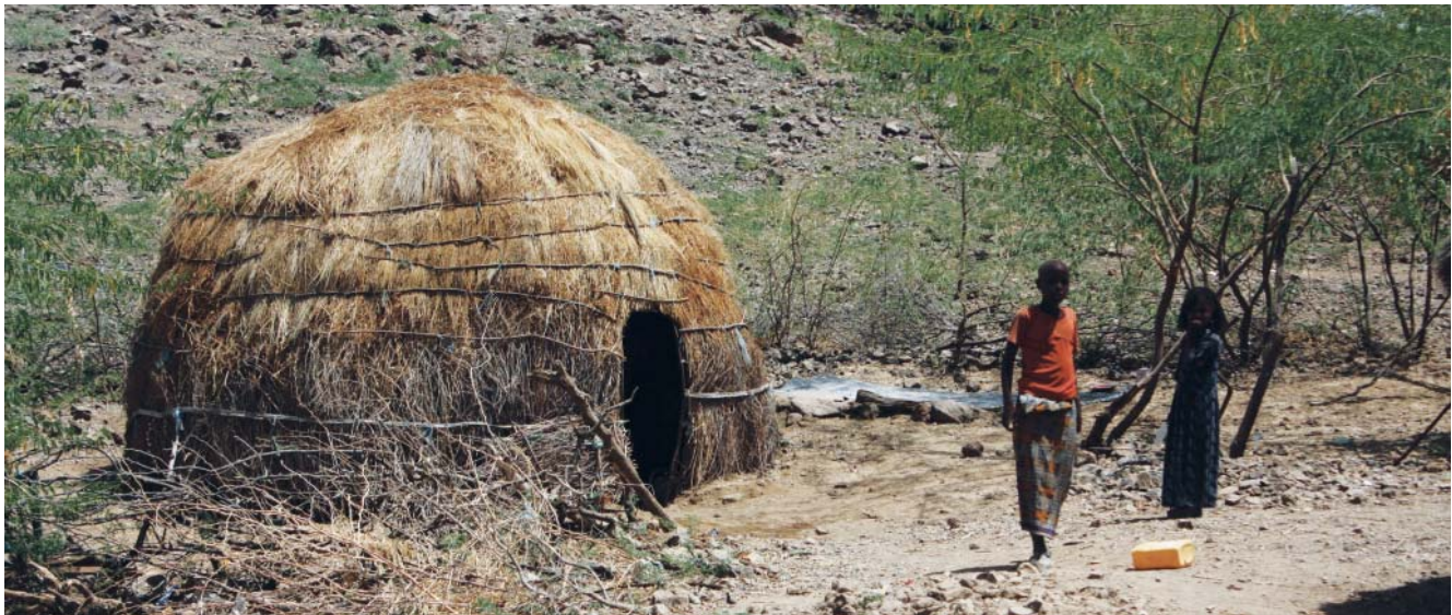
Fig. 212: Gubiyra, Yalo woreda : a free standing grass hut of a semi-sedentary family thatched with locally collected grasses
