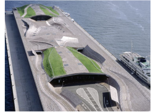
Abb.76: Yokohama Port Terminal
