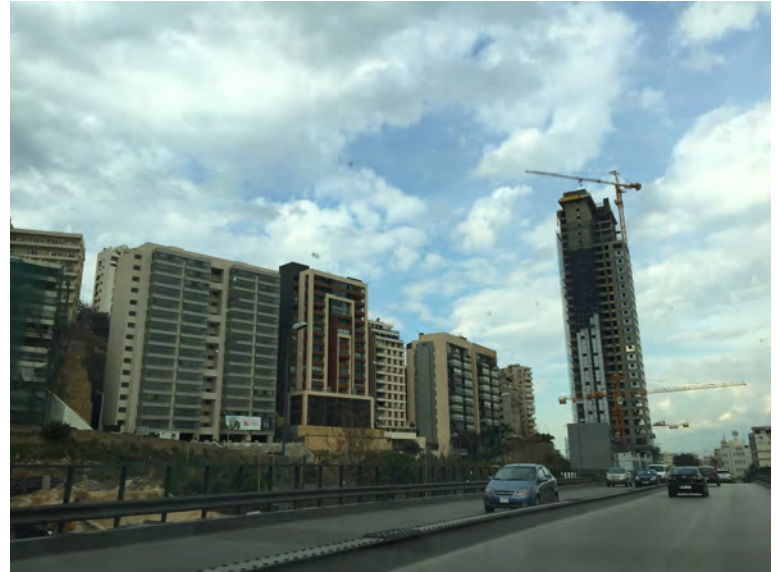
Abb.52: Bauboom in Beirut
