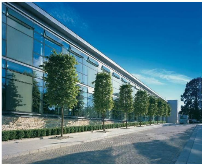
Figure 2.2.1&2.2.2: High-level windows for night-time ventilation in Wessex Water Operation Center Building in Bath, UK
