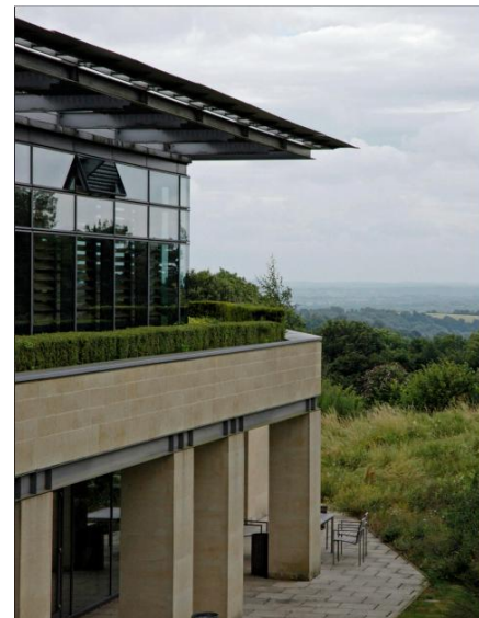
Figure 2.2.1&2.2.2: High-level windows for night-time ventilation in Wessex Water Operation Center Building in Bath, UK
