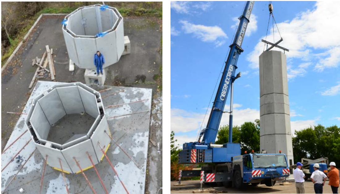
Figure 57. Prototype erection by using the innovative construction method [30]
