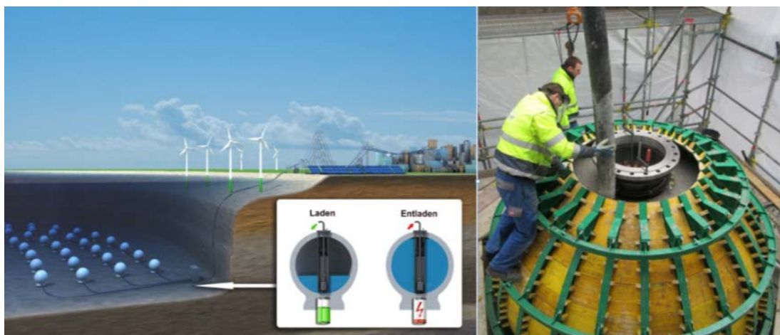
Figure 26. Storage of energy in concrete balls on the sea ground in Germany [26]
