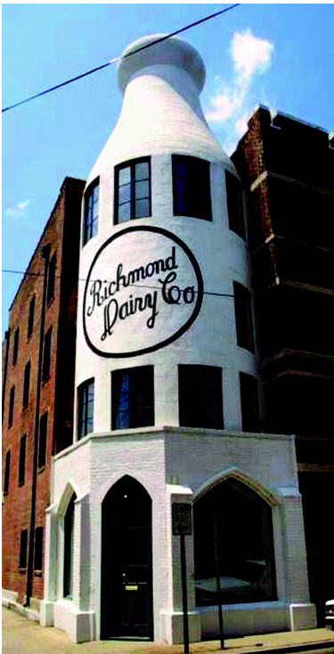
Abb.1.7, Richmond Dairy Co., Virginia
