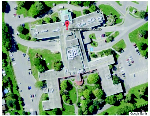
Abb.2.10, Newmarket Health Center, Kanada
