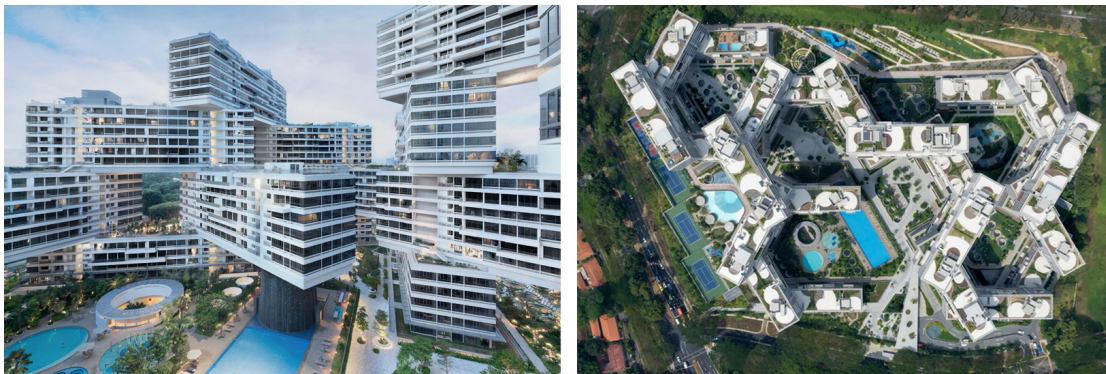
Figure 84: View from balcony and top view (buro-os.com, 2017)
