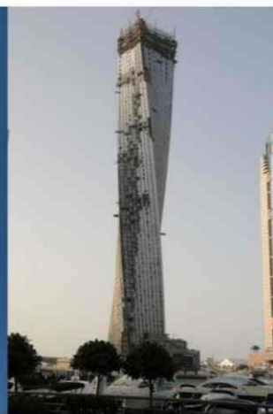
Abb. 25 Infinity Tower in Dubai
