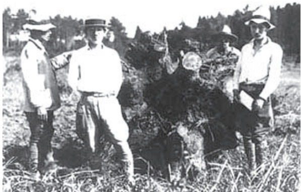
Img. 41: Dry conditions forced construction of the Hatori dam
