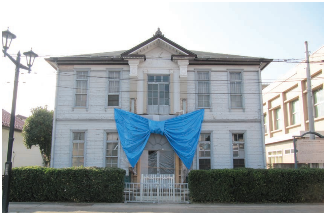
Img. 11: The 'House of Taisho Roman' in its reconstruction phase. The Blue Ribbon has become a sign of recovery for Yabuki town.
