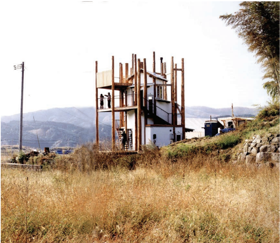
Img. 17: 'Home-for-All' after completion [ III ]
