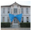
Img. 11 The 'House of Taisho Roman' in its re-construction phase. The Blue Ribbon has become a sign of recovery for Yabuki
