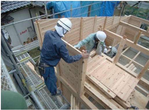
Img. 32: Constructing Core House in Itakura method
