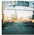
Img. 09 Destroyed shopping streets at Na- gata, Kobe after the Great Hanshin Earthquake in 1995
