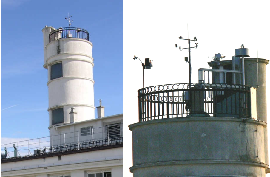
Figure 27: Roof mounted BPI weather station. Source: "Roof mounted BPI weather station" (2014)
