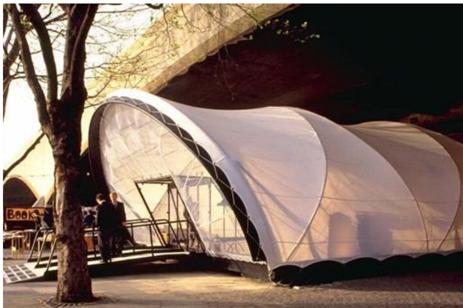
Figure- 46, a photo after montage of MOMI TENT
