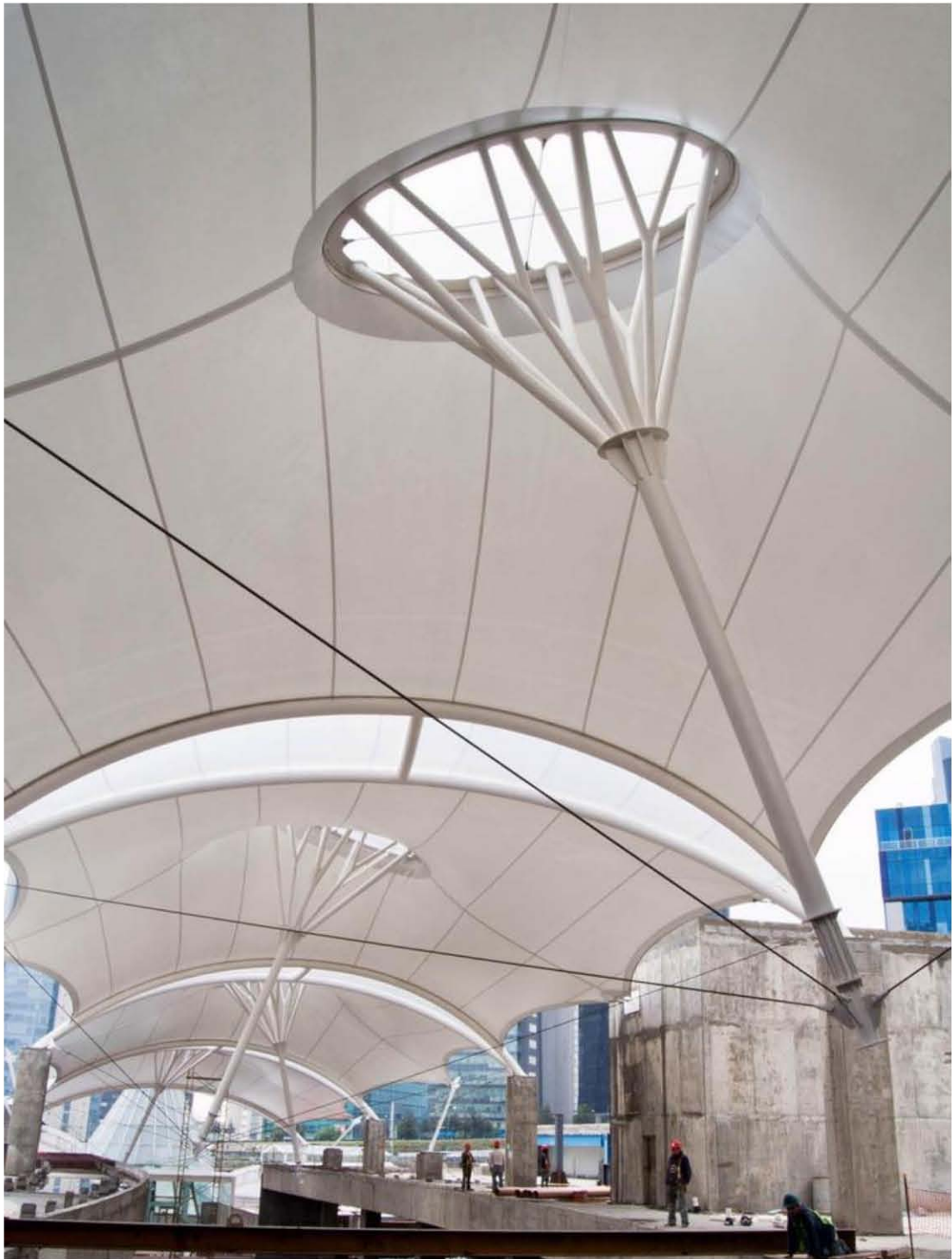
Fig. 26 – Example of branched central mast http://www.pinterest.com/pin/326018460496380651/
