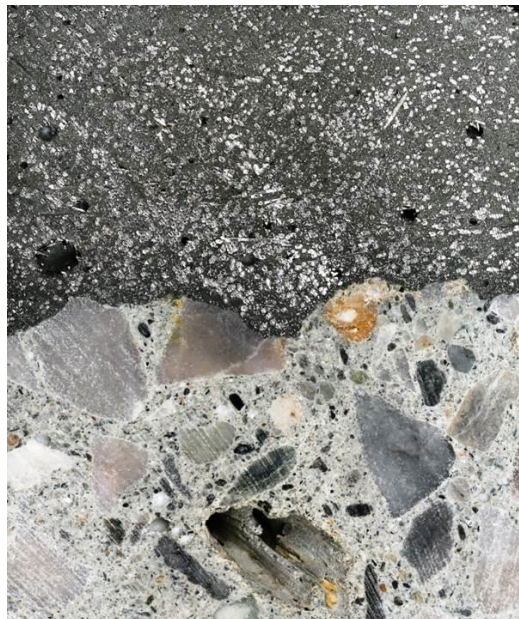
Figure 4.1: A layer of UHPFRC on top of an existing layer of concrete to display the differences in the composition of the materials (Brühwiler)
