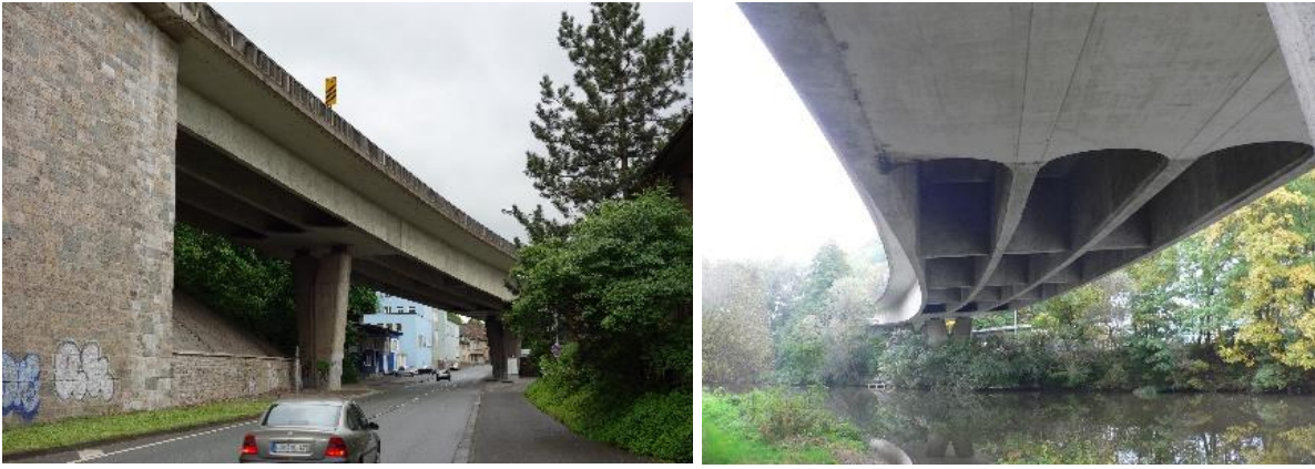
Figure 2.6: left: bridge over L3020; right: bridge over Lahn (Bösche & Curbach 2013a)
