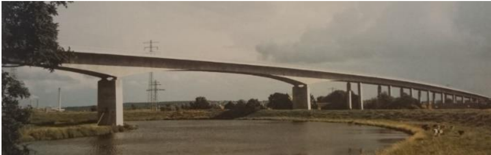
Figure 2.9: Stör Bridge near Itzehoe (Leonhardt 1982)
