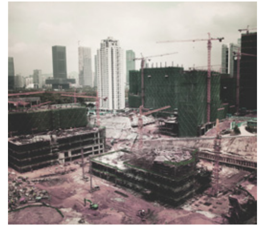
[pic19] Construction site of redevelopment in Gangxia, 2010
