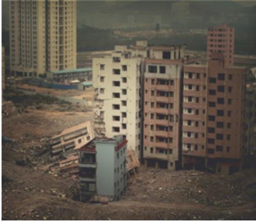
[pic16] Demolition of Gangxia's south-western part, 2010
