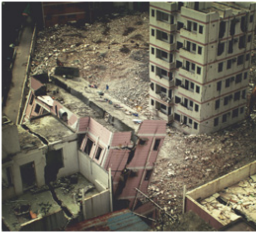
[pic17] Bulldozing the houses of Gangxia, 2010
