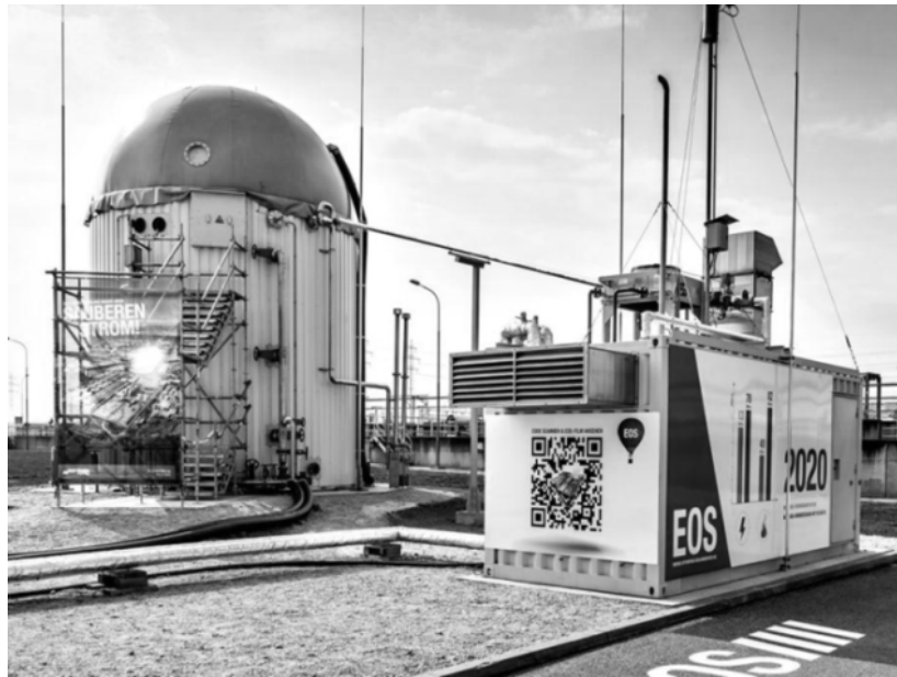
Fig. 6: Pilot plant for EOS project. Volume digester 130 m 3 , equipped with mechanical thickener, gas motor, reject water storage and treatment and complete sensor and control equipment
