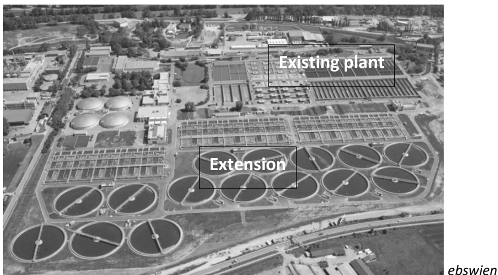
Fig. 2: Extension of the VMWWTP; start of operation 2005; the 2 nd stage is consisting of 15 lines with pre-denitrification tanks (mixed, rectangular) and 2 simultaneous nitrification/denitrification tanks with circular flow in series and a circular secondary sedimentation tank D = 64 m.
