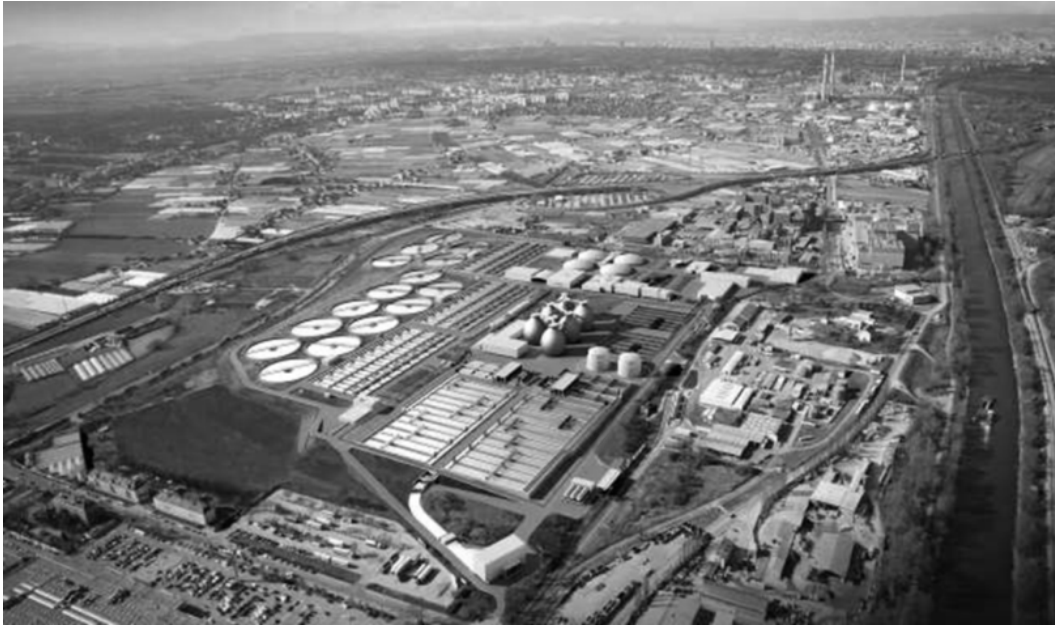
Fig. 5: Layout of the EOS Project, newly constructed primary sedimentation and first activated sludge plant in order to save space for 6 sludge digesters (12,500 m 3 each), gas motor station 2 gas holders, reject water nitritation and mechanical thickening
