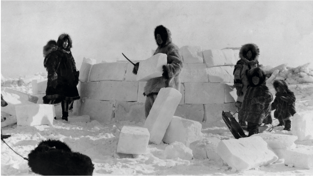
figure 47 - Inuit constructing an igloo with blocks of snow
