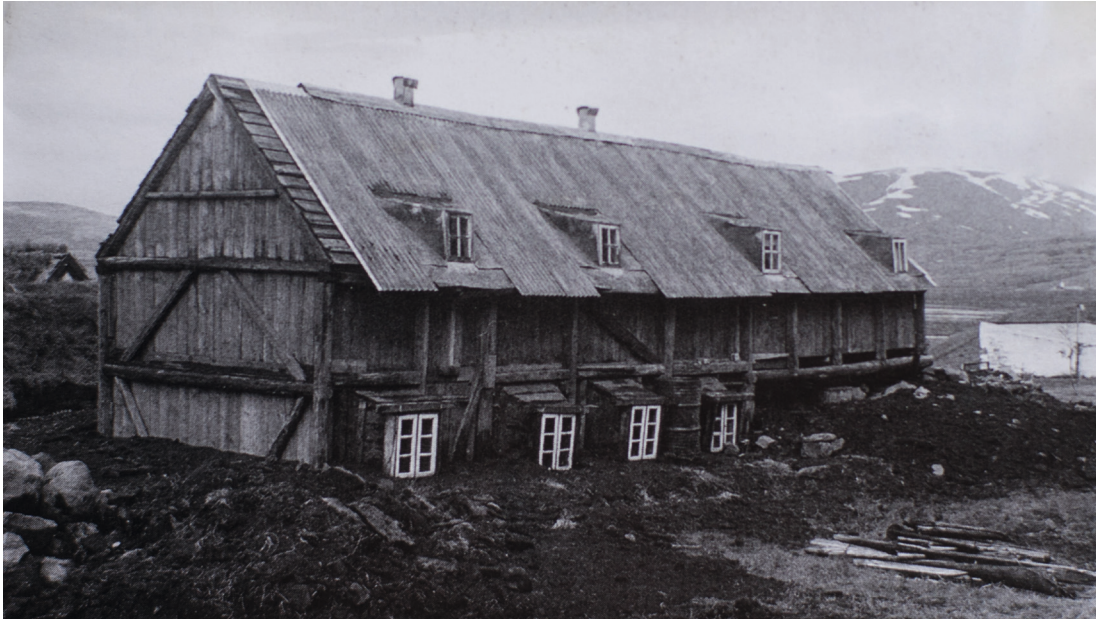
figure 41 - Baðstofa of Laufás turf farm stripped of its turf walls
