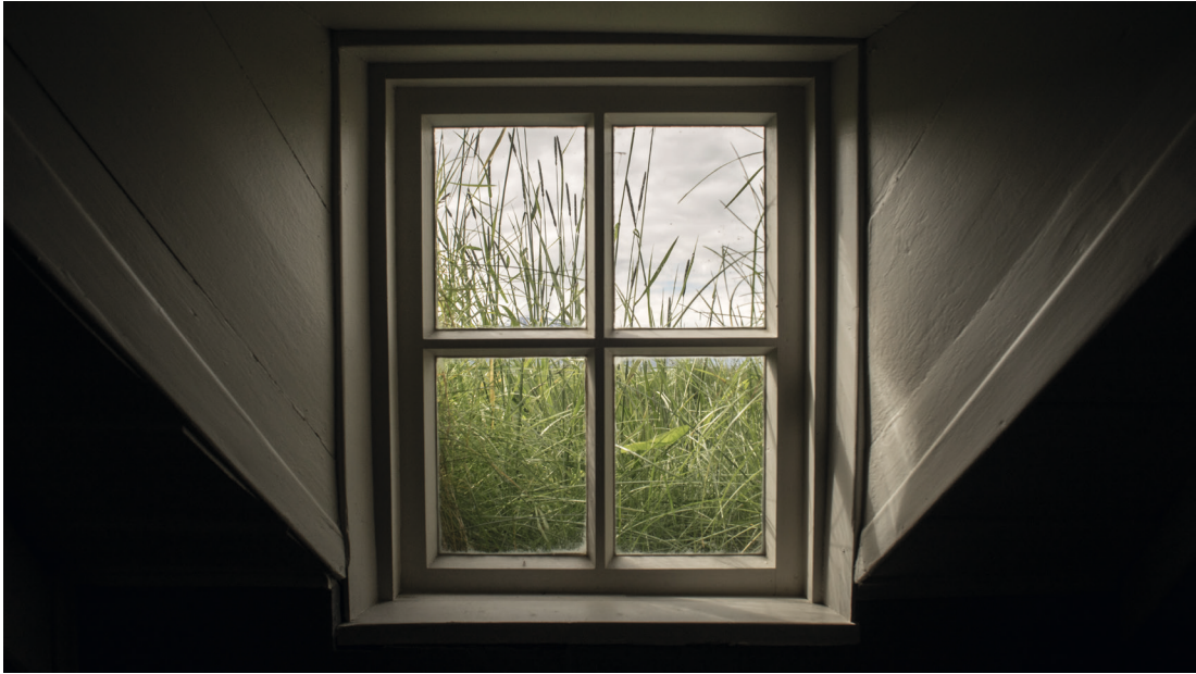
figure 54 - window detail from Laufás turf farm
