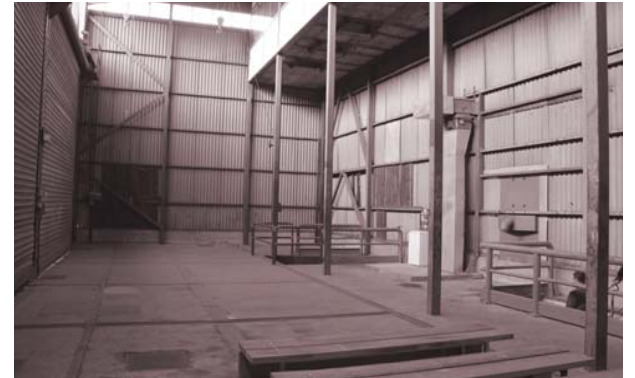
6 Fig.16 East station
