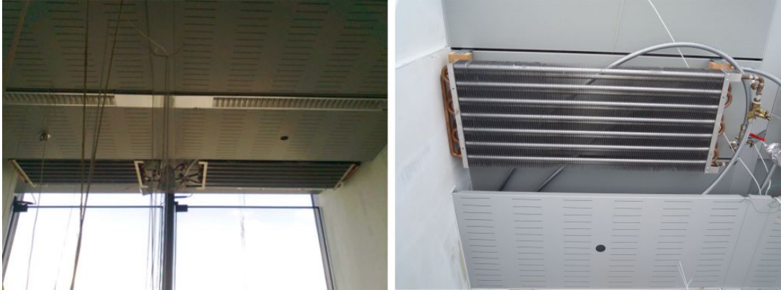
Figure 2.9: schematic overview - additional cooling element
