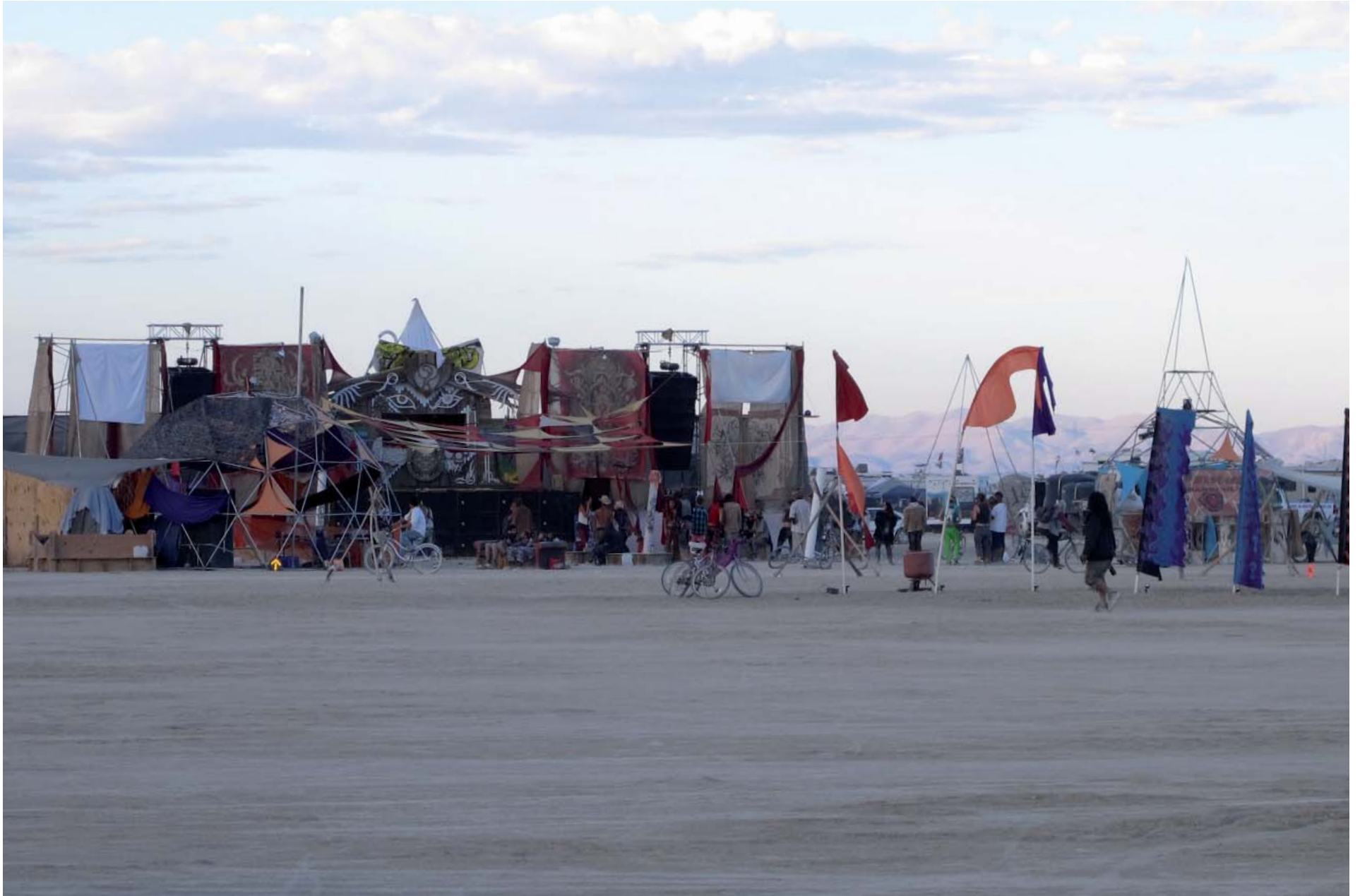
Figure 48: Construction at Burning Man 2012
