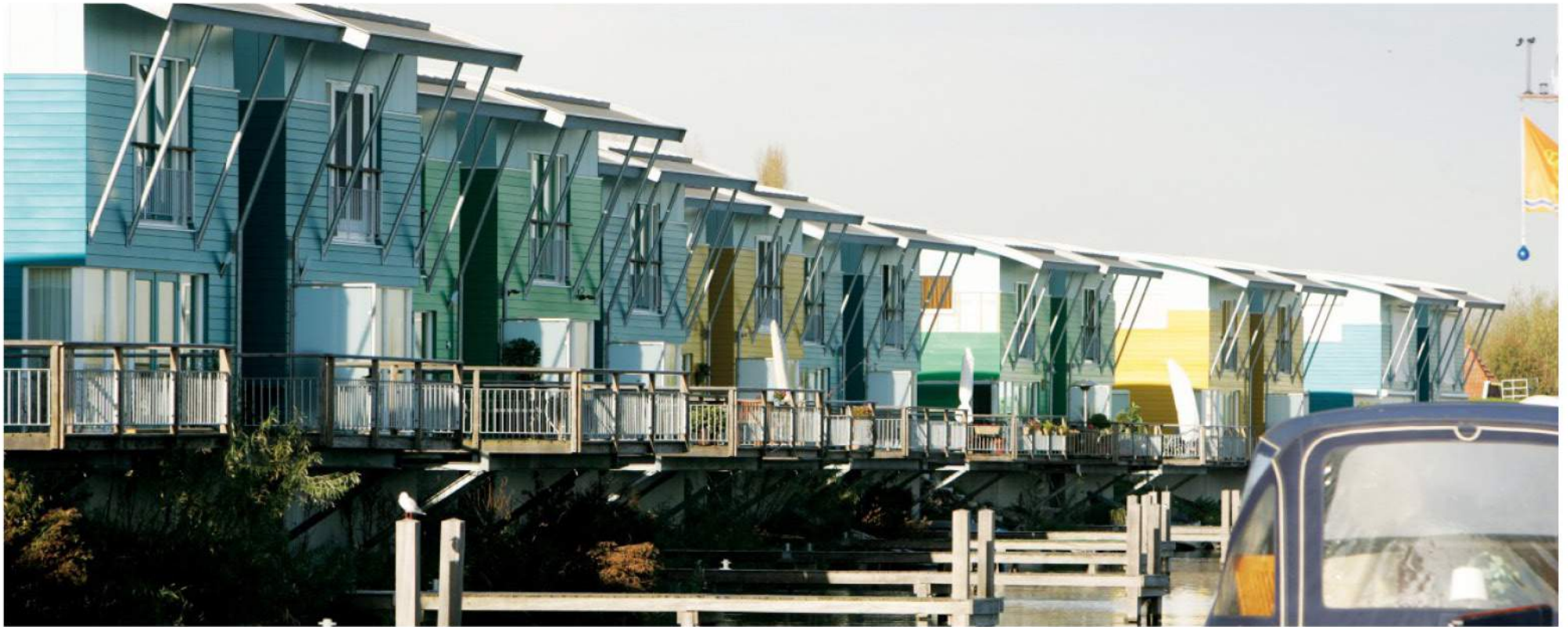
Figure 68 | Amphibious housing in Maasbommel, Netherlands
