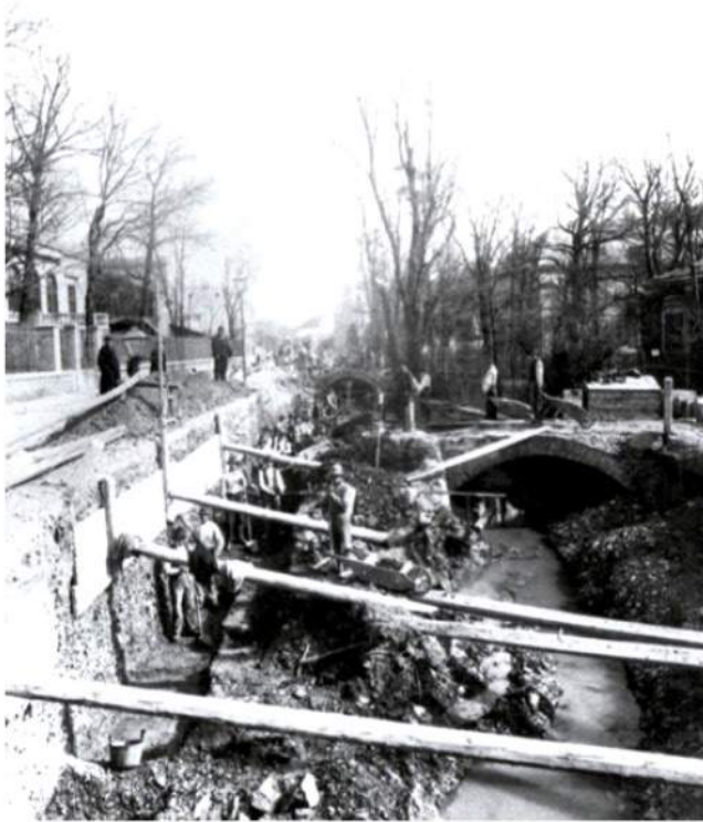
Figure 13 | Channel construction in the neuwaldegger street in the former Neuwaldegg municipality, starting in 1884
