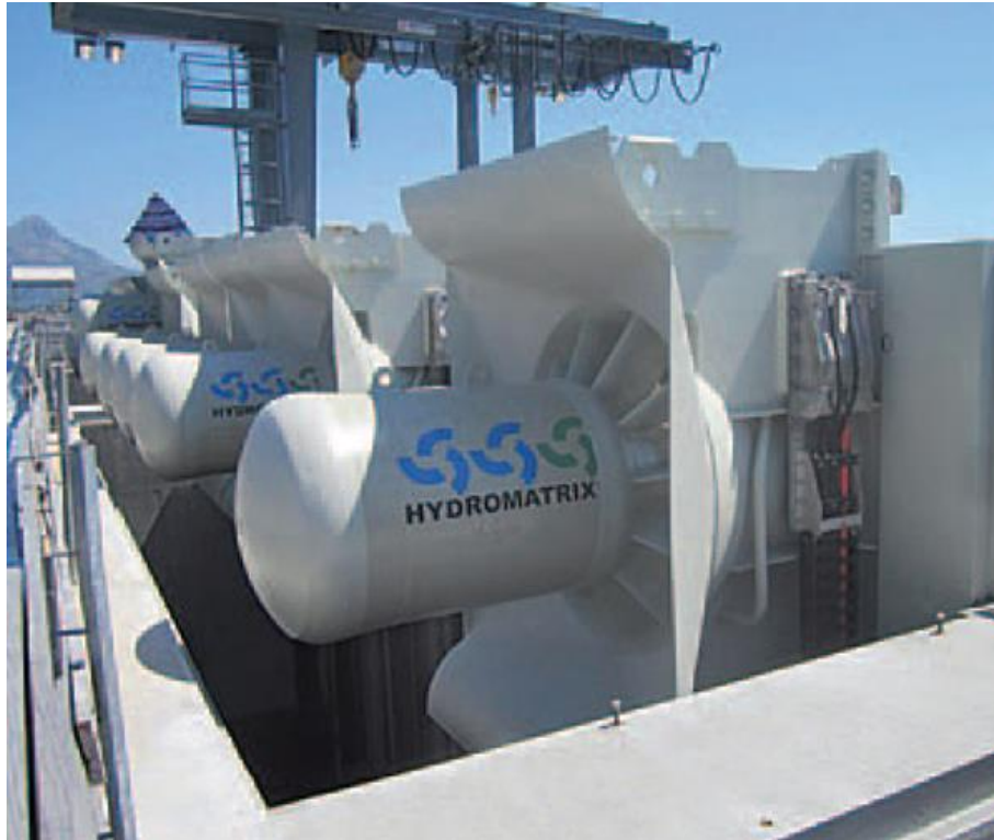
Abb. 4.8 Ashta Kraftwerk, Shkoder, Albania [6]
