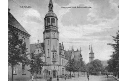
19 Main Post Office (1899-1901)
