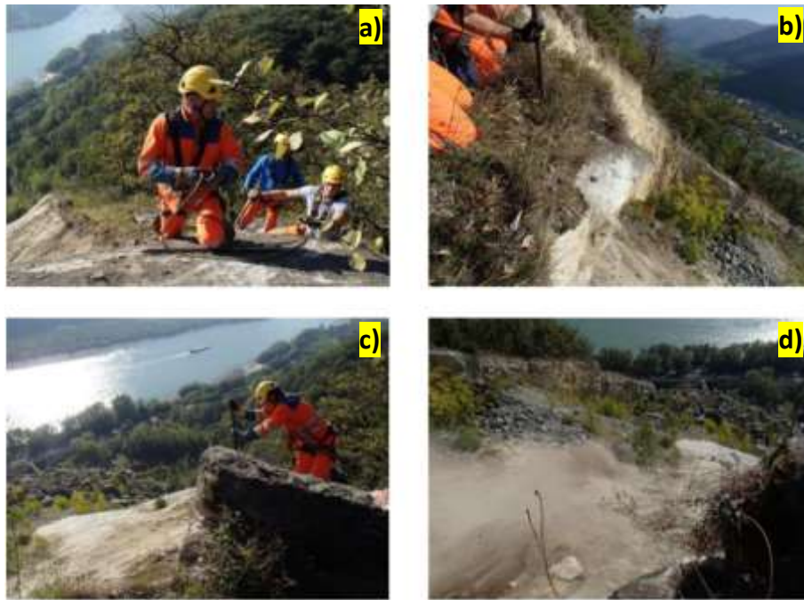
Figure 8.5. Triggering of rockfalls and rockslides on the top quarry area by the troops of the local construction management.
