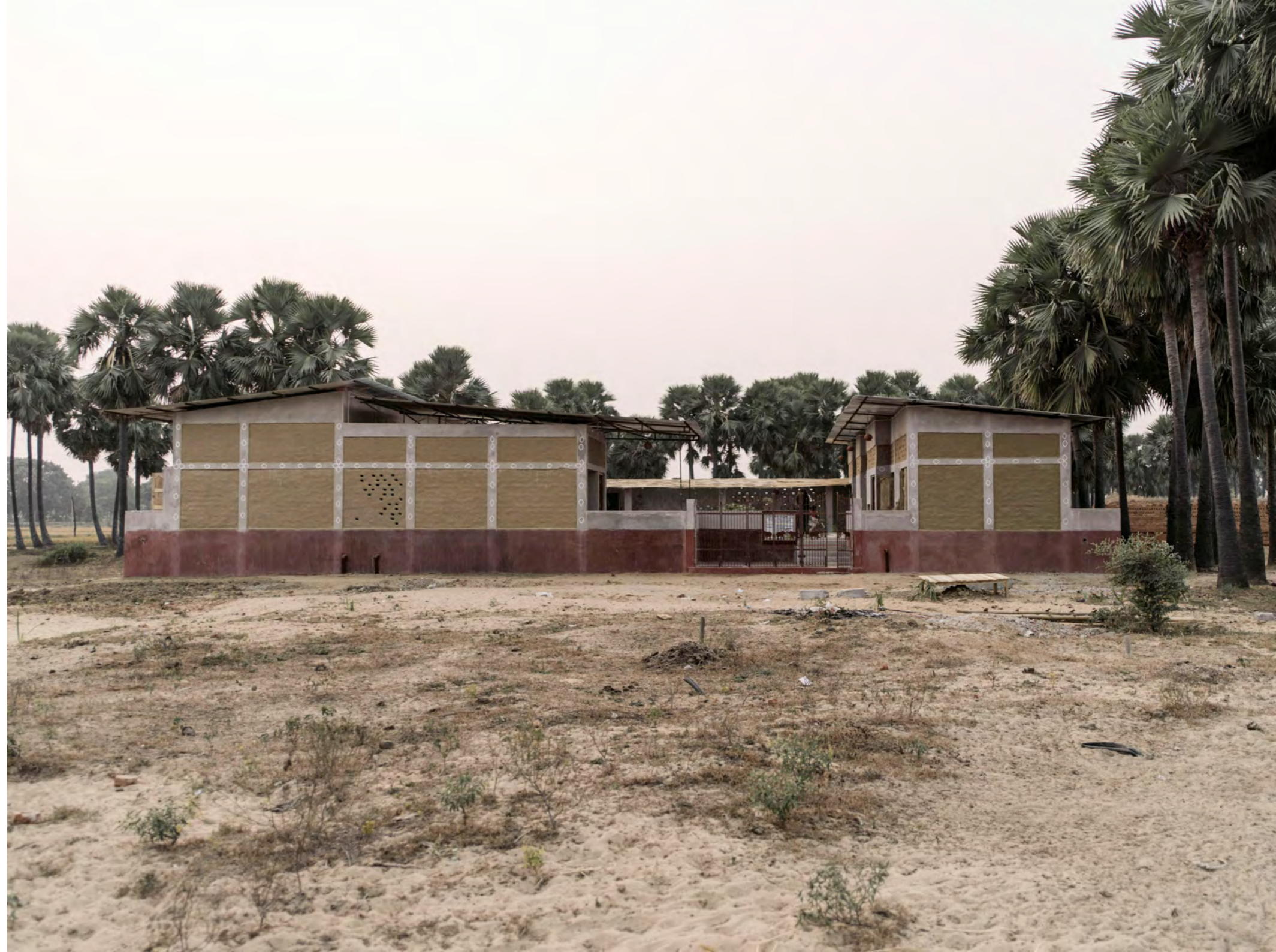
Front view of the ready school
