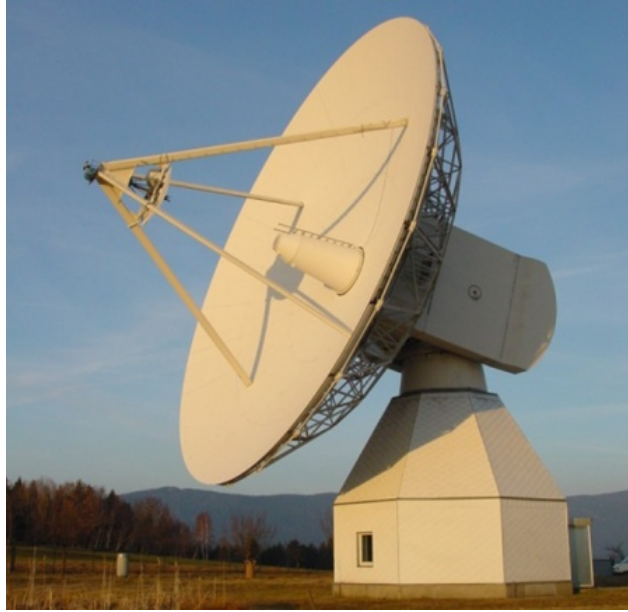
Figure 1.1: The paraboloidal reflector with the subreflector and the feedhorn of the 20 metre diameter telescope in Wettzell, Germany [Heinkelmann, 2013].
