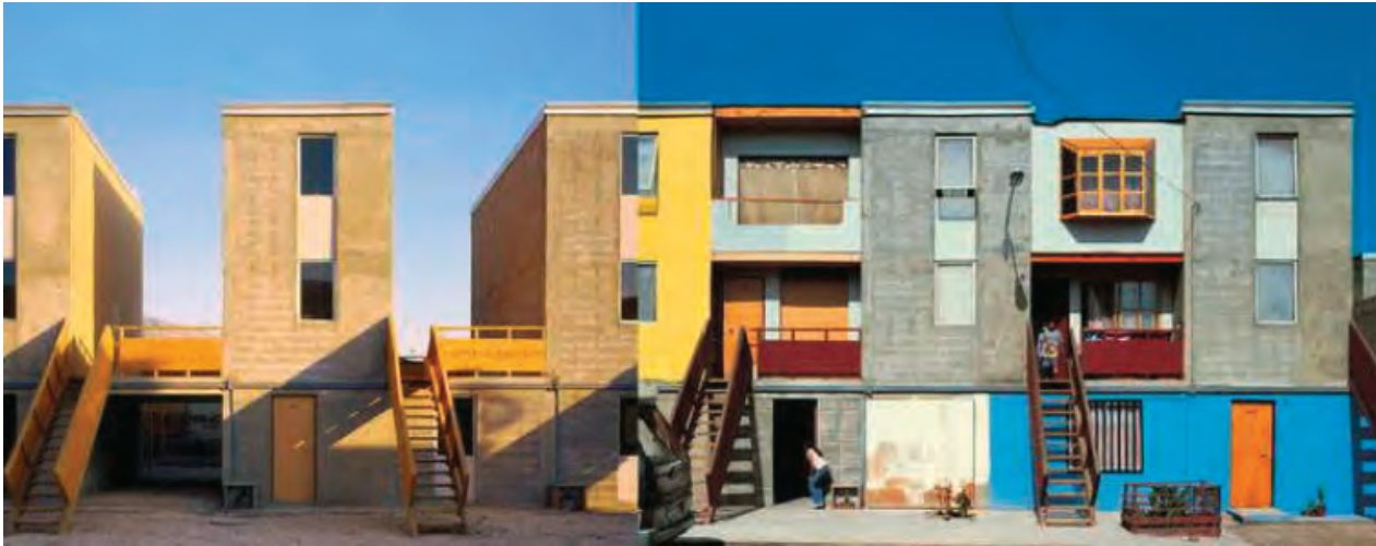
Before and after upgrading https://www.studyblue.com/notes/note/n/arc-001-study-guide-2010-11-ncarb/deck/9736673 (07.01.2016)
