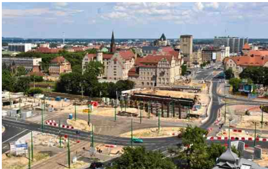
Fig. 39. The Kaponiera Rounabout under construction
