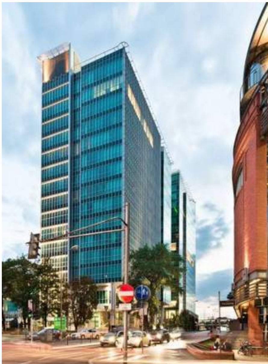
Fig. 34. Poznań Financial Center and Andersia Tower
