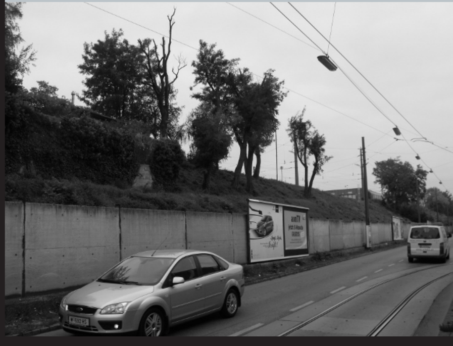
fig. 22: the Avedikstrasse - the building site on the left
