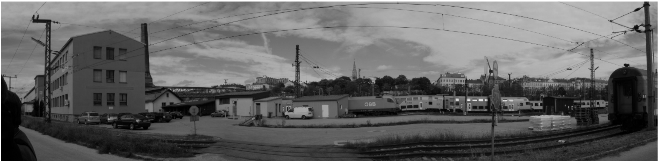
fig. 26: repair and assembling shops of the Austrian Federal Railways close to the building site
