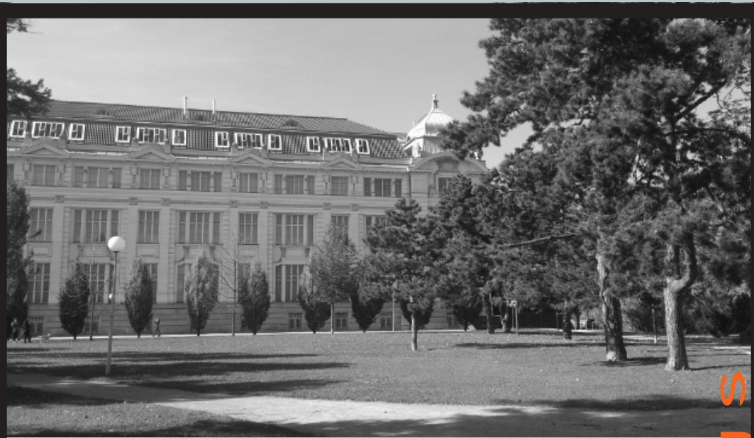
fig. 20: view from the park next to the museum and opposite the building site
