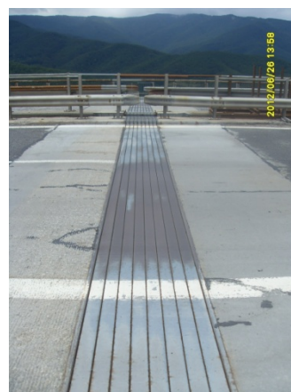
Abb. 60: Dilatationsfuge
