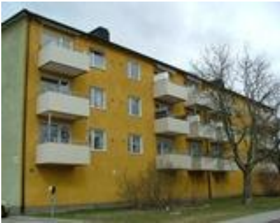
Figure 4-13 Photo of the multi-family house in Sweden which is used as a reference building in the case study
