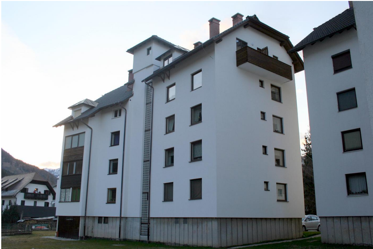
Figure 4-18 Photo of the multi-family house in Slovenia which is used as a reference building in the case study
