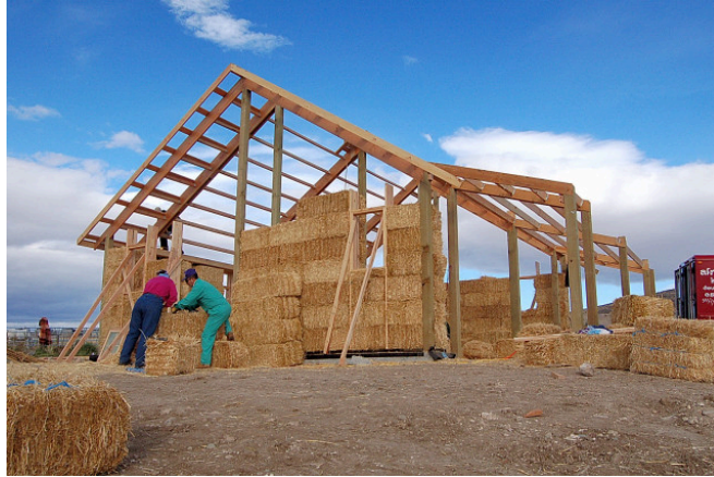
Figure 7: Infill method, Ellensburg workshop (2007)
