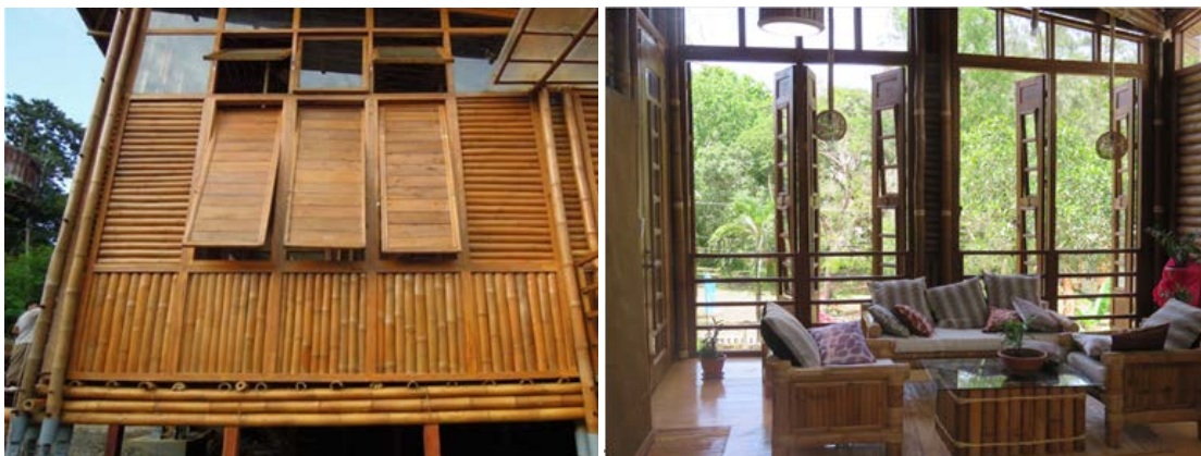
Figure 7: Shutters at the southwest corner; big openings at the building's east side
