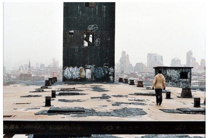
Image 28: The roof of the Red Hook Grain Terminal
