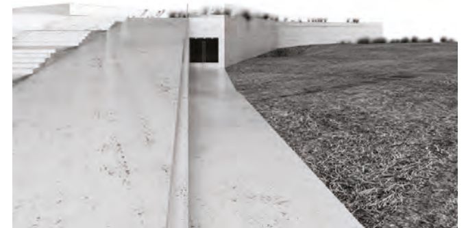
Ill. 62 Entrance and ramp to the rooftop
