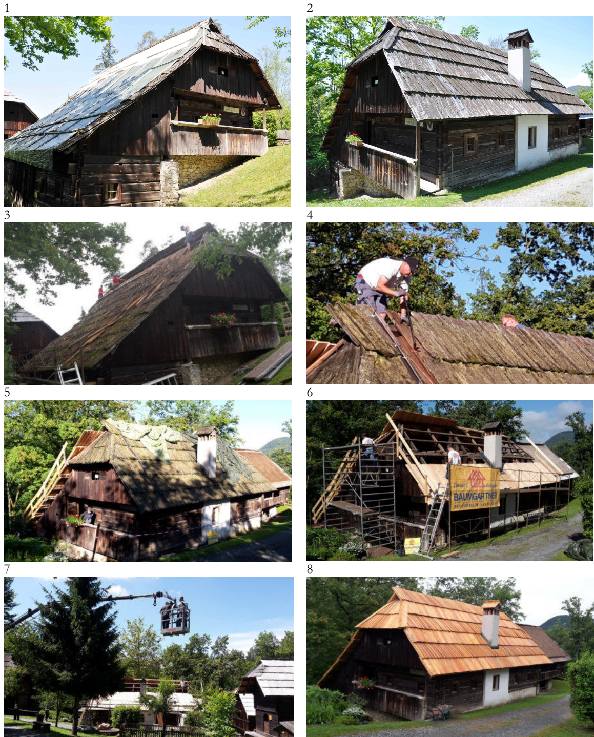
Fig. 3.98. The sequence of the Urchhaus's roof renovation (Courtesy of Maria Saal Freilichtmuseum, retrieved on 22 March 2017)
