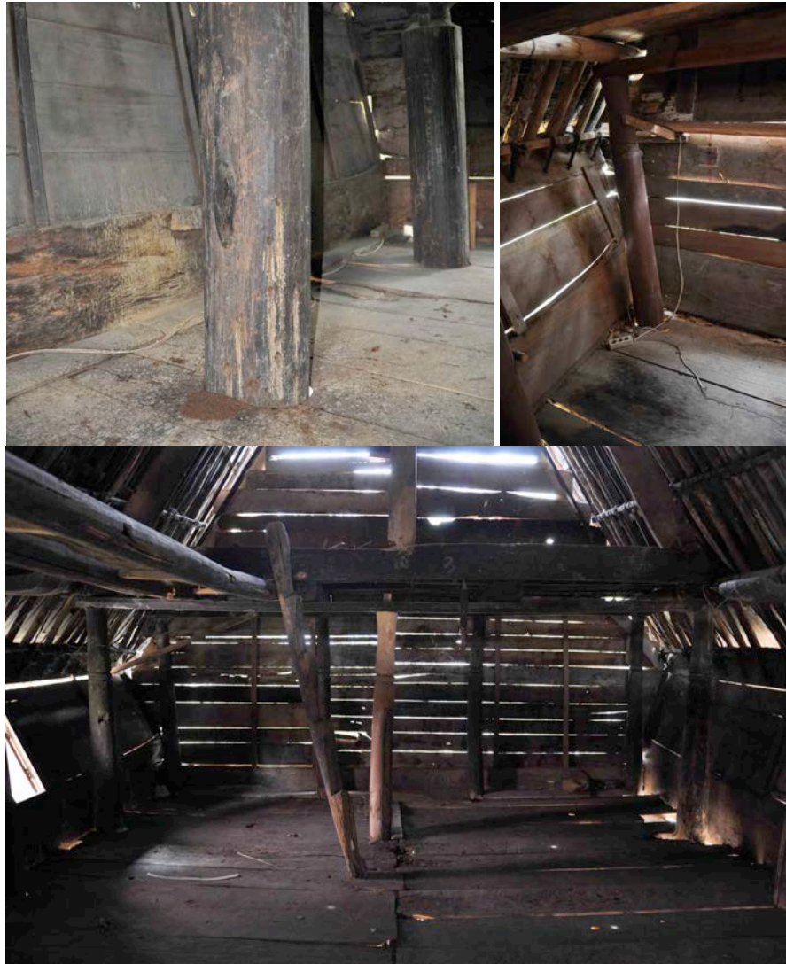
Fig 5.25. Some weathering situations in TBSC; at Sopo number 3 (top left) and at Ruma number 3 (top right) and at Ruma number 1 (below) (Source: author)
