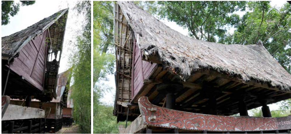
Fig 5.15. Harsh condition with decayed fibers roof at the oldest Sopo (number 4) (Source: author)
