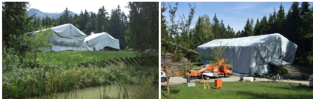
Fig. 3.95. Chemical treatment process in Salzburger Freilichtmuseum (Courtesy of Salzburger Freilichtmuseum)
