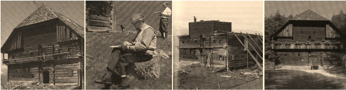
Fig. 3.7. In situ Säuerling; recording the house in May 1964; dismantling the house in June 1964; relocated house at Stübing in 1965 (left to right) (Courtesy of Stübing Freilichtmuseum from Pöttler)
