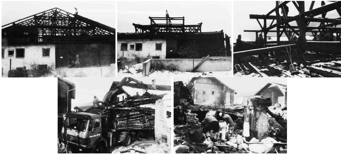
Fig. 3.87. The sequence in dismantling the house (left to right) (Courtesy of Tiroler Bauernhöfe Kramsach Freilichtmuseum)
