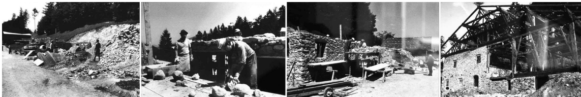
Fig. 3.88. The sequence in re-erecting the house (left to right) (Courtesy of Tiroler Bauernhöfe Kramsach Freilichtmuseum)
