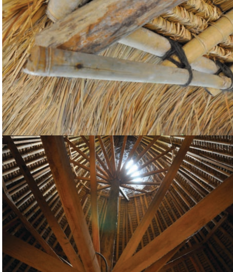
Fig 5.20. Some modern modification; Bamboo nailed at rafter (top) Square wooden beams encircling central pole of Mbaru Niang (below) (Source: author)
