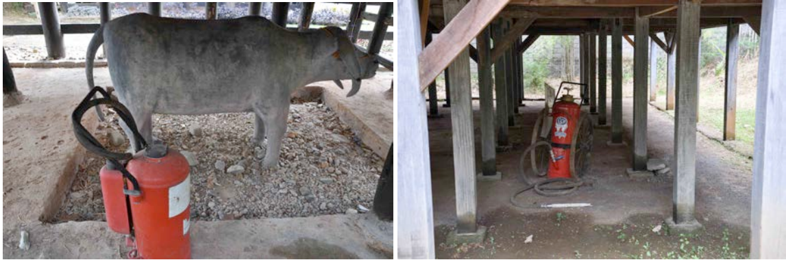
Fig 5.22. Carelessly placement of fire extinguisher beneath a Ruma in TBSC (left) and beneath Palembang house in Taman Nusa (right) (Source: author)
