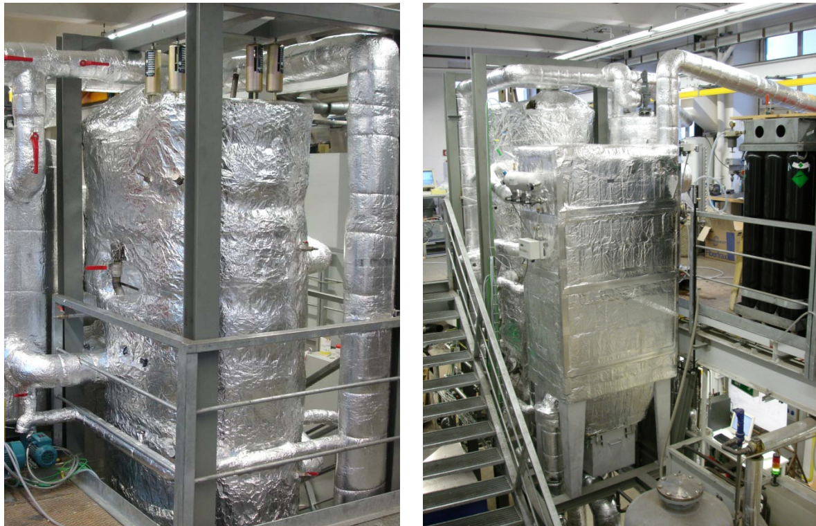
Figure 1.2: 140 kW chemical looping combustion plant at Vienna University of Technology
