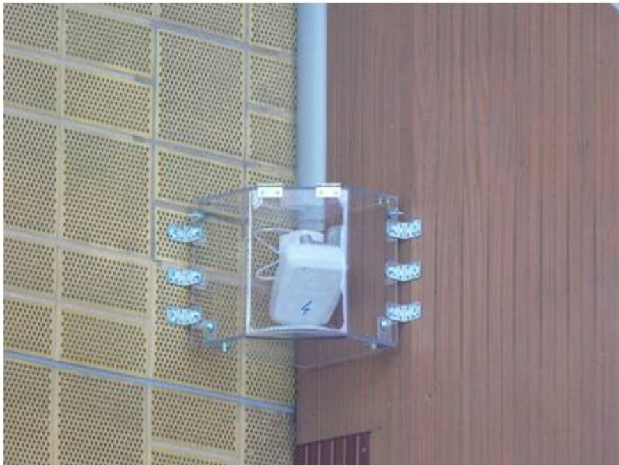
(a) Installed signal receiving sensors (base stations) in the corners of a university's sports hall.
