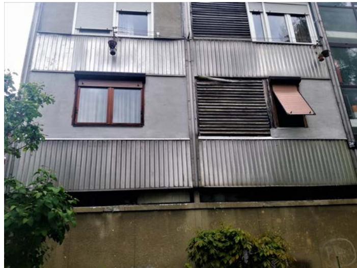
Figure 9 Partial renovations of the façade (Photo collection of the author)
