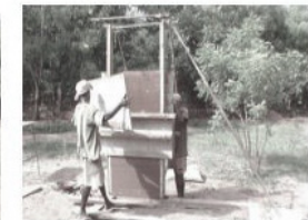
Lifting panels of the first form to the third one
