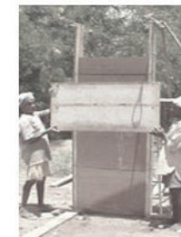
Lifting panels of the second form to the fourth one
