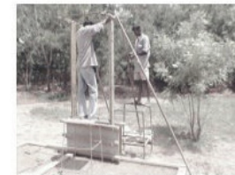
First panels and adjusting the end shutters
