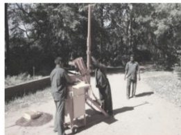
Pushing back the hopper to level the soil in the mould
