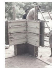
Adjust panels of the third form of a corner wall
