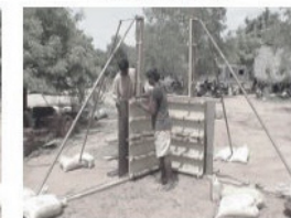
Adjusting panels of the second form of a corner wall
