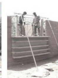
Ramming a long wall in the second form
