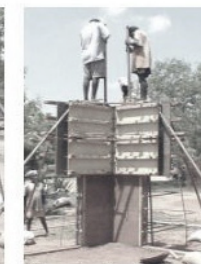
Ramming the fourth form of a corner wall
