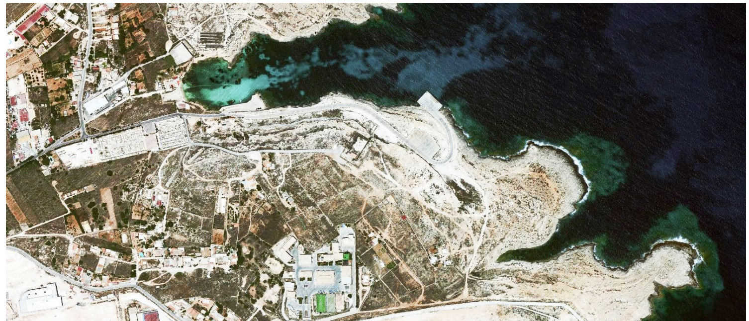
Fig. 5.03 Lampedusa: Cala Pisana, Cala Uccello - the construction site
