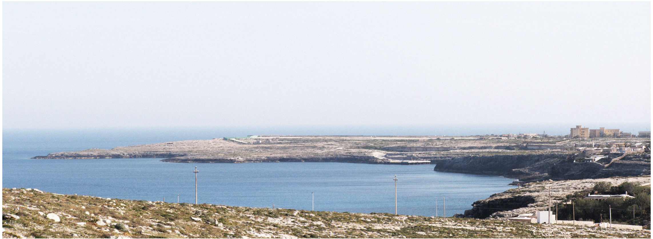
Fig. 5.05 view on the construction site from the Northern coast
