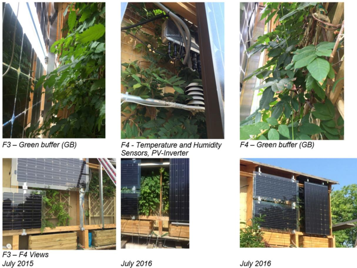
**Fig. 7.** F3–F4 GB – pictures. Above: inside of the GB and view of the GF behind both types of PV-modules, semitransparent and standard. Below: comparison of the plants evolution in one year and outside view.
